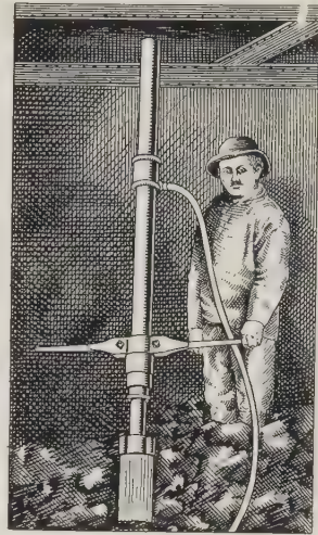
FIGURE 264 — Hydraulic spade for clay used in the Forth bridge caissons.
