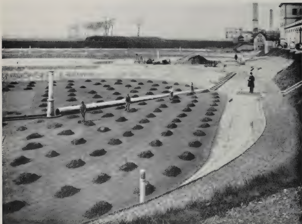
B. Cleaning a slow sand filter at the Hampton works of the Southwark and Vauxhall Water Company, c 1890. After draining the water from the filter, the top layer of sand, up to about an inch thick, was scraped off and removed by hand. (p 563)
