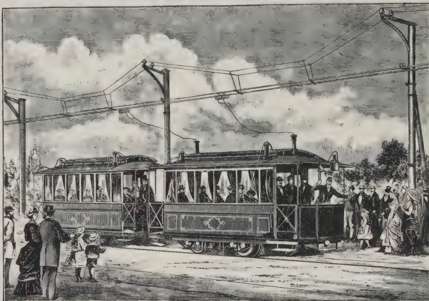
FIGURE 181—Electric line between Frankfurt-am-Main and Offenbach, 1884, by Siemens & Halske. The leading car had a single driving axle to which the motor was geared down. The overhead conductor- and return-lines consisted of slotted gas-piping in which ran shuttle-shaped runners with lugs projecting downwards through the continuous slot and attached by light frames and cables to the car.
