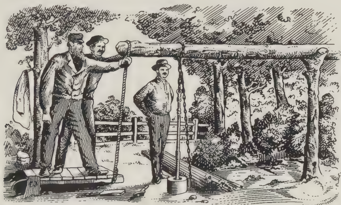
FIGURE 40—'Kicking down' a well by the spring-pole drilling method.
