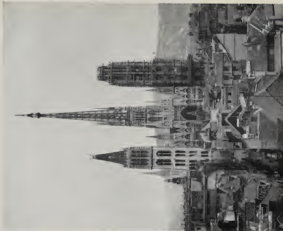
B. The cast iron spire of Rouen Cathedral, built 1876. (p 472)
