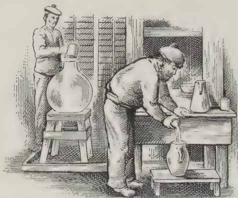
A stage in the manufacture of mercury fulminate at Westquarter, Scotland, c 1890.
