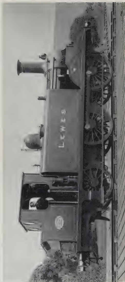
C. Lionlin, Brighton, and South Coast Railway engine, the 'Lewes', one of William Stroudley's famous 'D' class, the first of which was built in 1873. (p 326)
