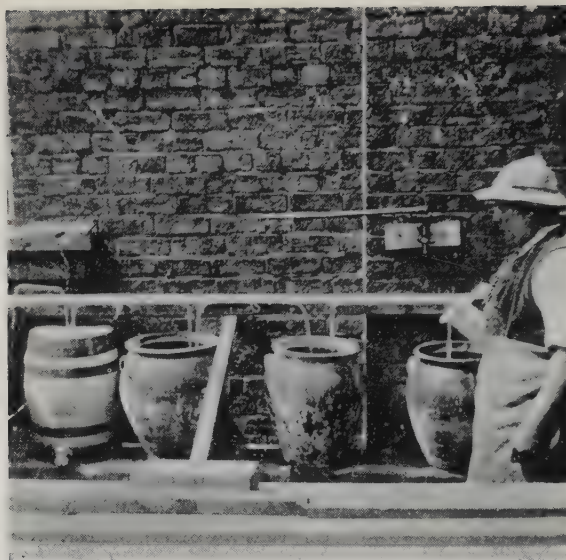
A. The first regular chlorination of a British water supply, at Lincoln, in 1905. A solution of sodium hypochlorite was made up in the stone jars and fed into the water. (p 567)
