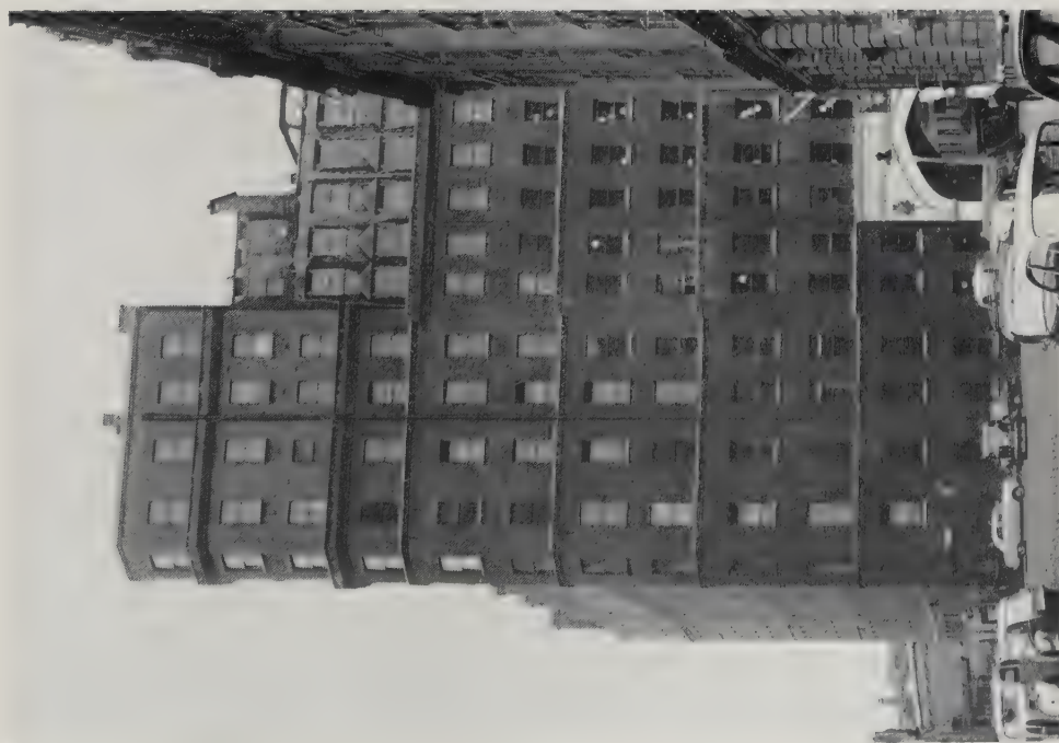
A. Queen Anne's Mansions, London's first skyscraper. Building was begun in 1873, with brick walls and for the most part fire-resisting concrete floors. (p 478)
