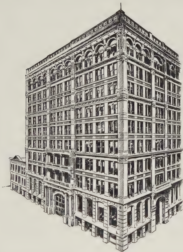
FIGURE 254— The Home Insurance Building, Chicago, an early example of the use of Bessemer steel in building.
