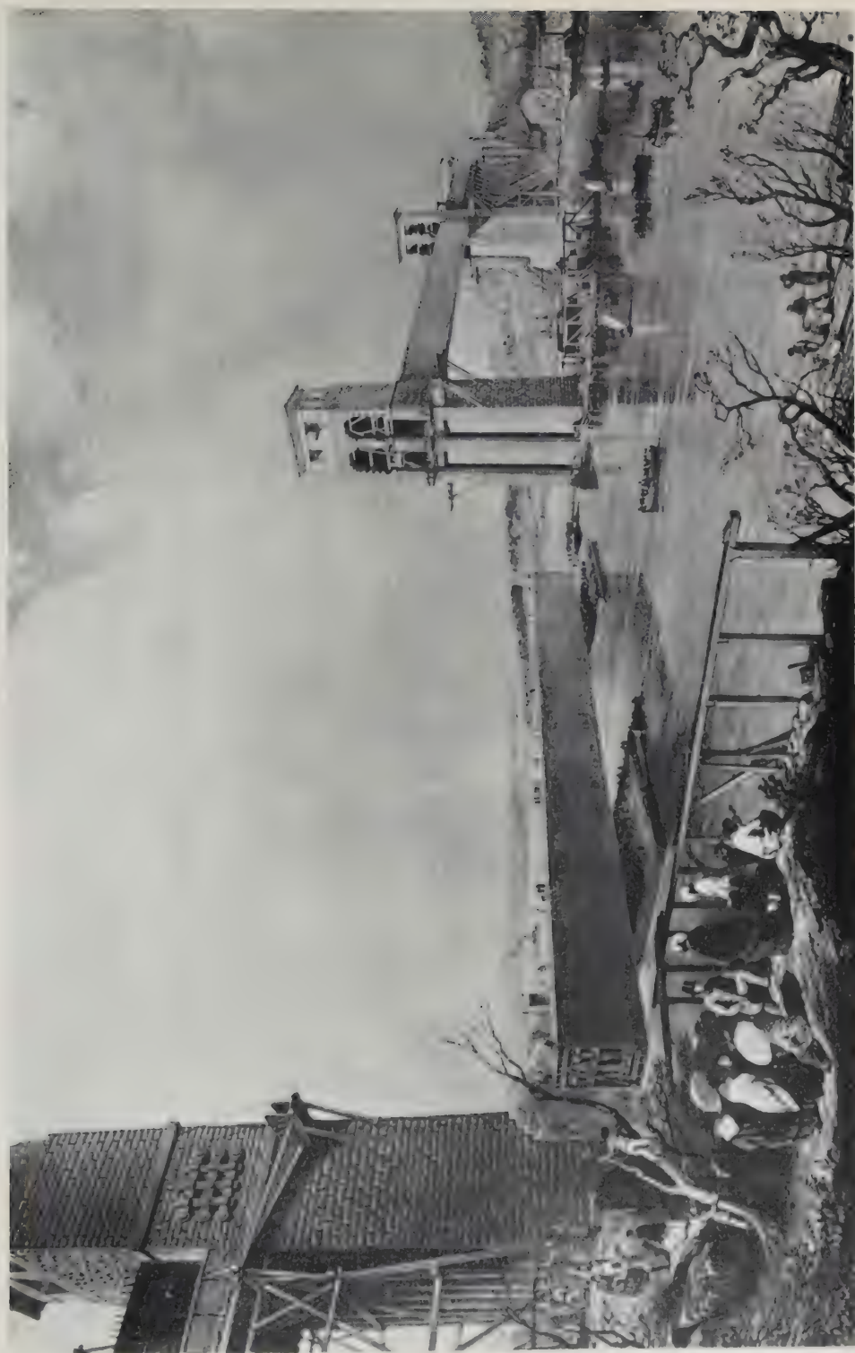
One of the 450-ft tubes of the Britannia bridge being floated into position, 1849. (p 504)
