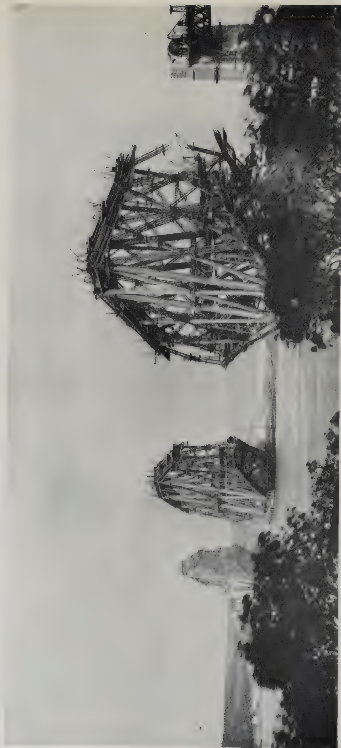
Erection of cantilevers proceeding on the Forth bridge, c 1890. (p 307)
