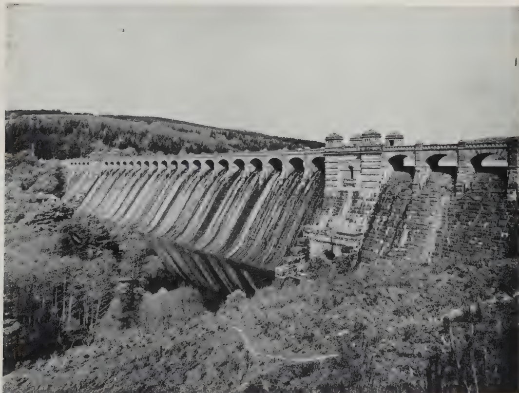
B. Vyrnwy Dam, north Wales, built 1881-91. The dam is 1172 ft long at the crest, and has a maximum height from foundations to water level of 144 ft. It impounds a maximum of 12,131 m gallons of water. (p 557)
