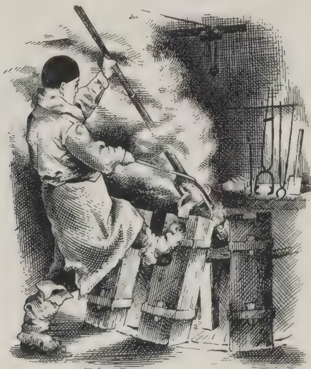
FIGURE 320—Casting brass ingots in iron strip moulds.
