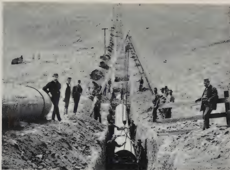
A. A 44-in riveted steel water-line as installed at San Francisco, 1885. The line is in service at the present time. (p 559)
