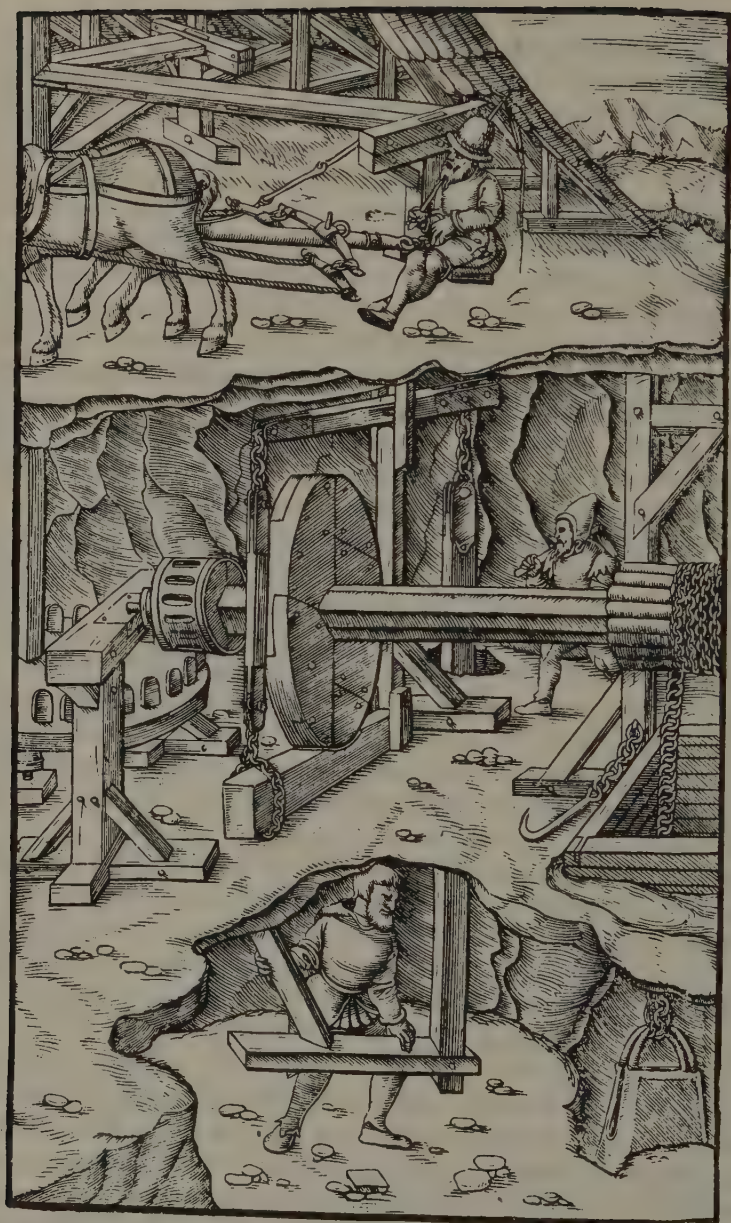
FIG. 44. Use of horse-whim in mining. Agricola, 1556
