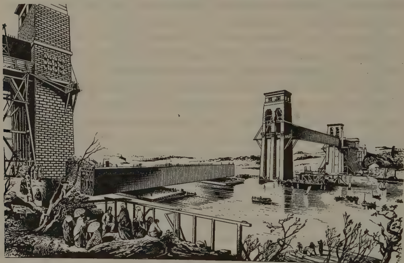
FIG. 227. One of the 459-ft tubes of the Britannia bridge being floated into position, prior to raising, 1849
