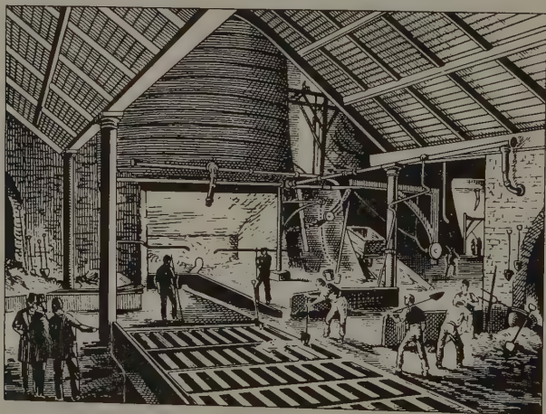
FIG. 242. Running molten iron into pigs, c. 1850
