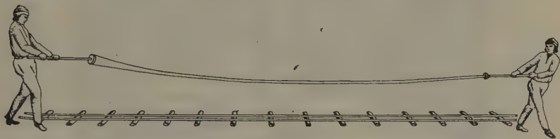
FIG. 293. Drawing glass tubing, preparatory to laying it on the 'ladder'
