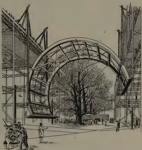
FIG. 202. Raising the first ribs of the transept roof of the Crystal Palace, 1850
