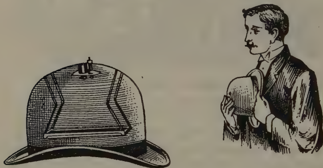
FIG. 330. 'Detective' camera concealed in the crown of a hat, 1891
