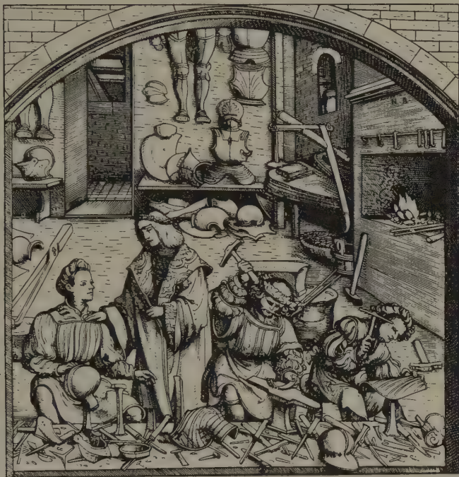
FIG. 48. Armourer's workshop of the early sixteenth century, showing some of its products and the tools used in making them
