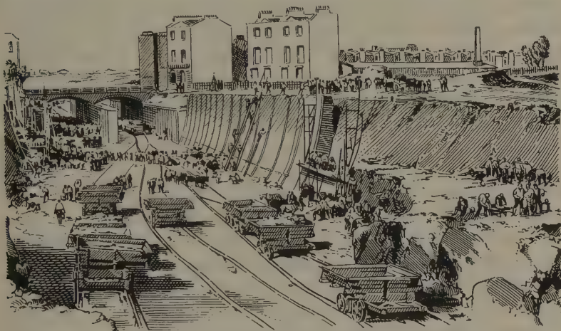
FIG. 223. Building of retaining wall at Camden Town station, London, 1837
