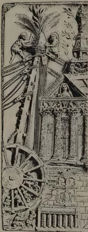
FIG. 112. Crane powered by tread-mill, from a Roman carving, c. A.D. 100
