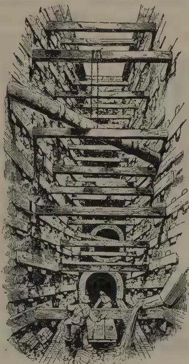
FIG. 213. Deepening a sewer under Fleet Street, 1845
