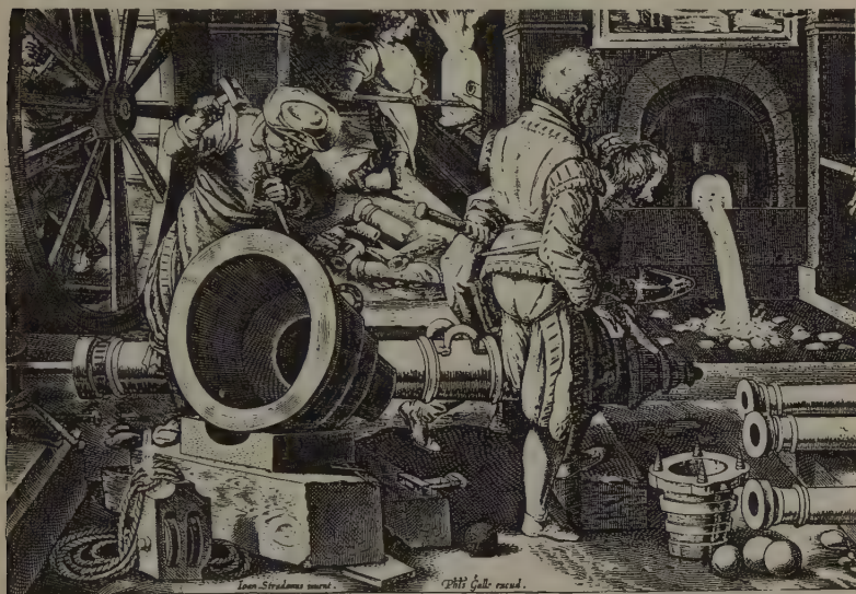
FIG. 46. Foundry for casting bronze cannon, with power supplied by treadmill, sixteenth century
