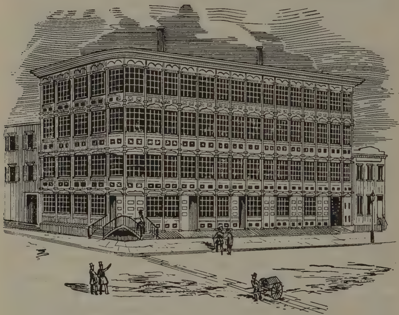
FIG. 201. Building with cast-iron frame, New York, 1851
