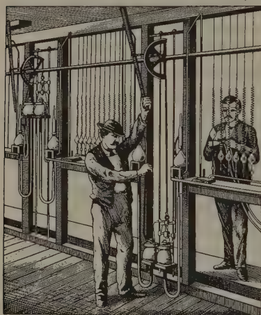
FIG. 317. Evacuation of electric lamp bulbs with a mercury air-pump, c. 1883
