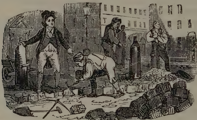
FIG. 216. Paving a London street with setts of Scottish granite
