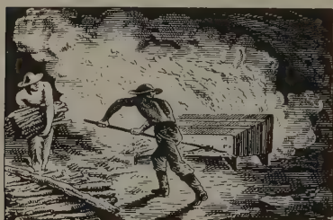
FIG. 249. Heating rocks preparatory to splitting them by throwing on water
