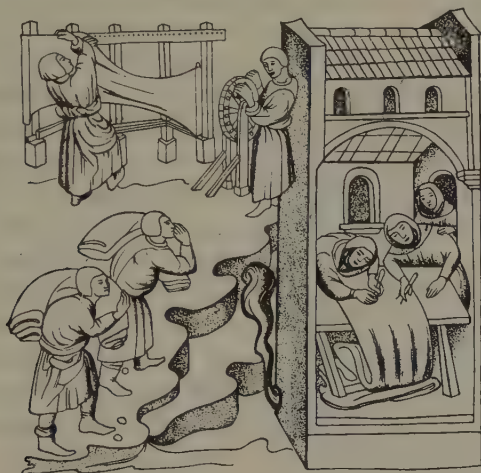
FIG. 35. Cloth finishing in a monastery: ( right ) correcting faults; ( left ) stretching on a tenter-frame. From an Italian manuscript of 1421
