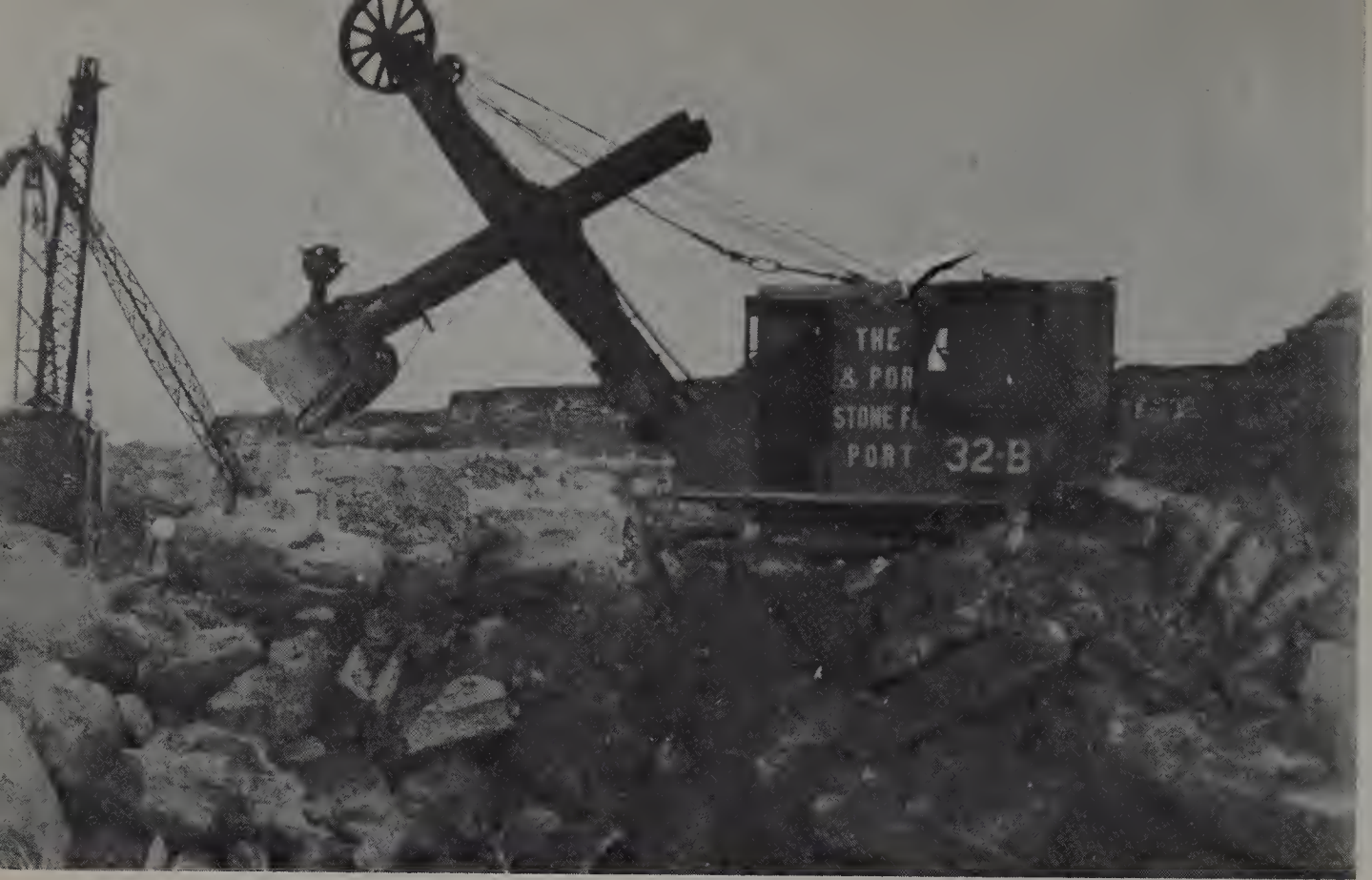
Ruston & Hornsby steam navvy removing overburden at Portland quarries, c.1910
