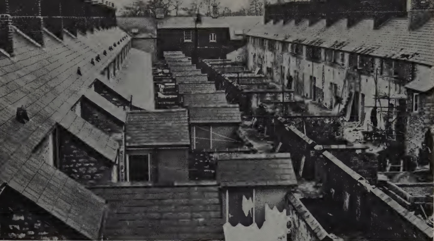
Houses in the Railway Village during modernisation (1960s). Work on the houses at the left of the picture has been completed. At the back of the terrace on the right the old wash-houses and outdoor privies have been demolished, but the new outbuildings have not yet been started
