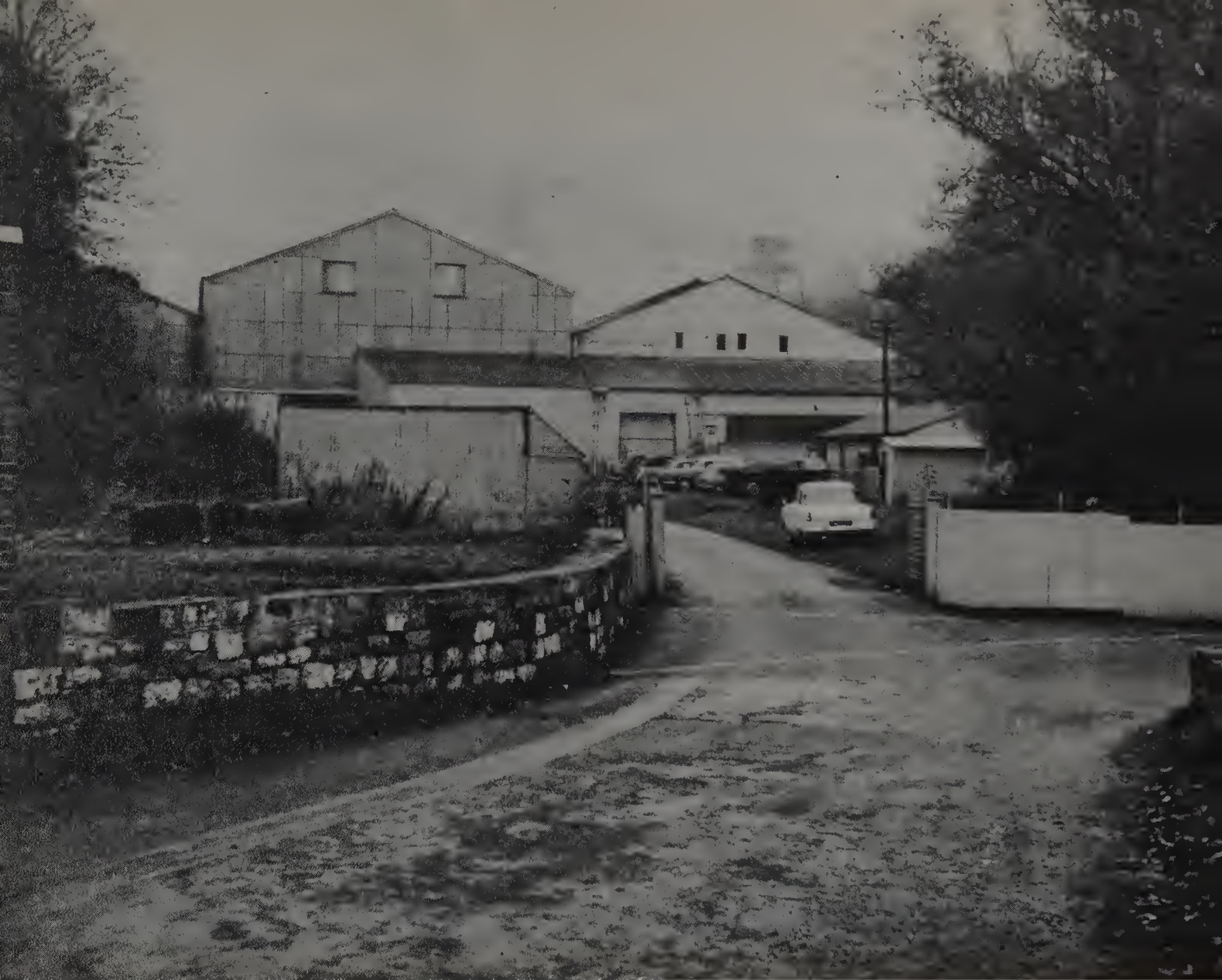
Tinplate Works (now closed), Redbrook, Forest of Dean. The dark-coloured blocks in the wall are copper-slag, evidence of a previous era of metal-working on the site
