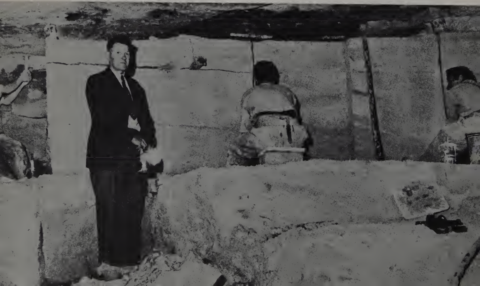
Monks Park Quarry: hand-sawing blocks at face
