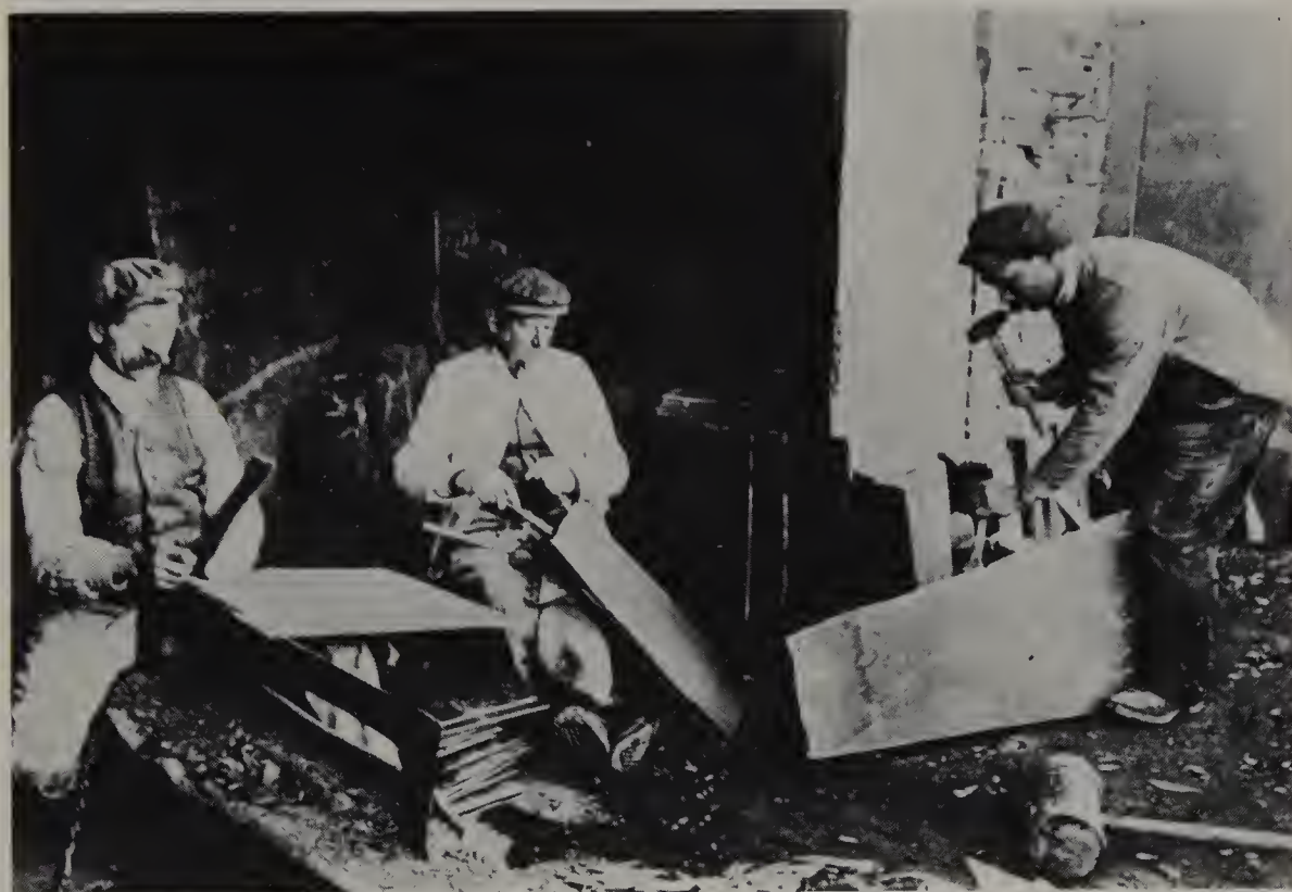
Splitting and trimming roofing-slates at Dinorwic, c.1890
