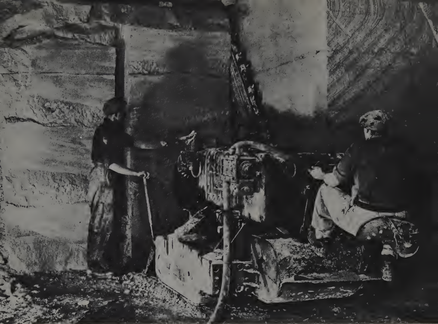
Monks Park Quarry: cutting out limestone blocks with converted 'Samson' coal-cutting machine
