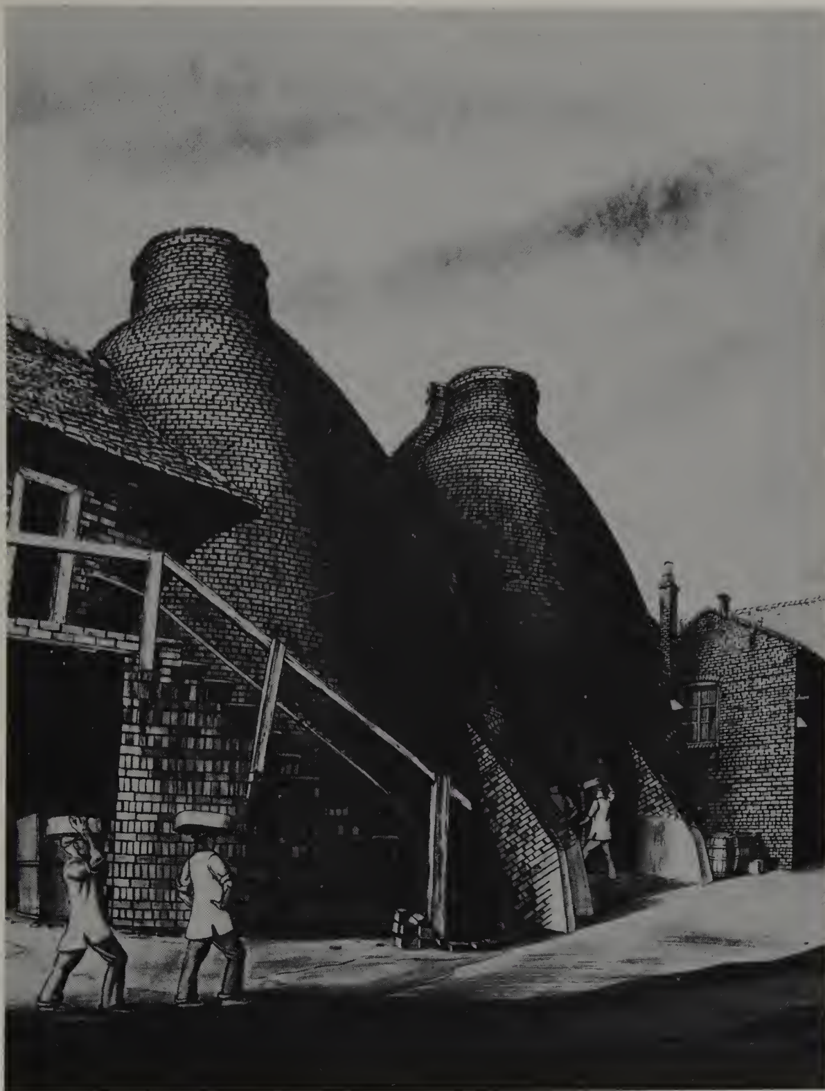
Bottle kilns at Etruria ( c. 1769), now demolished. The drawing, by L. G. Brammer, shows men carrying saggars of pottery into the kiln
