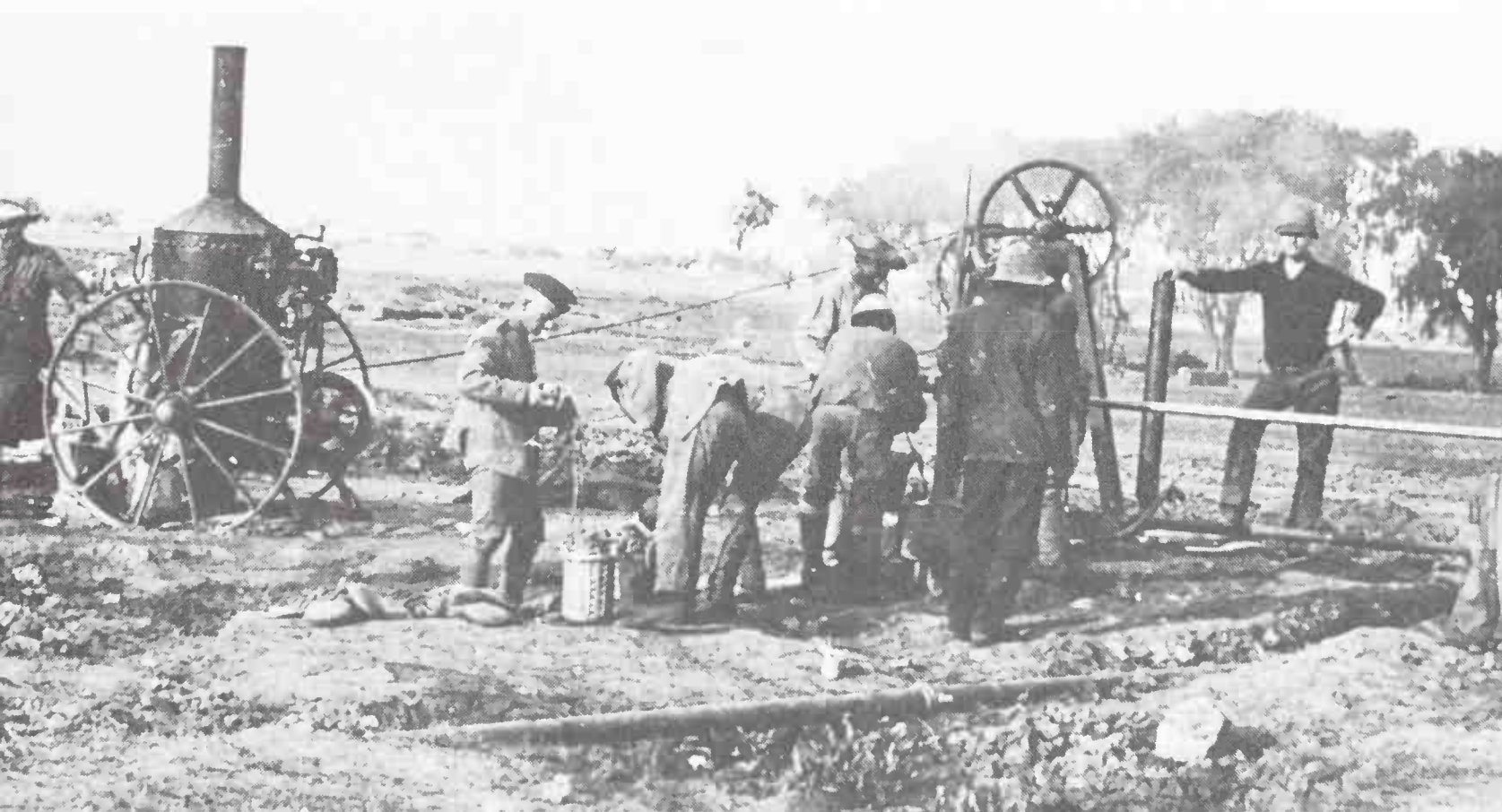
Beating enteric: Steam pump, sterilizing unit and newly laid pipes at the Portland hospital, all part of the army's answer to the high death rate during the Boer War.
