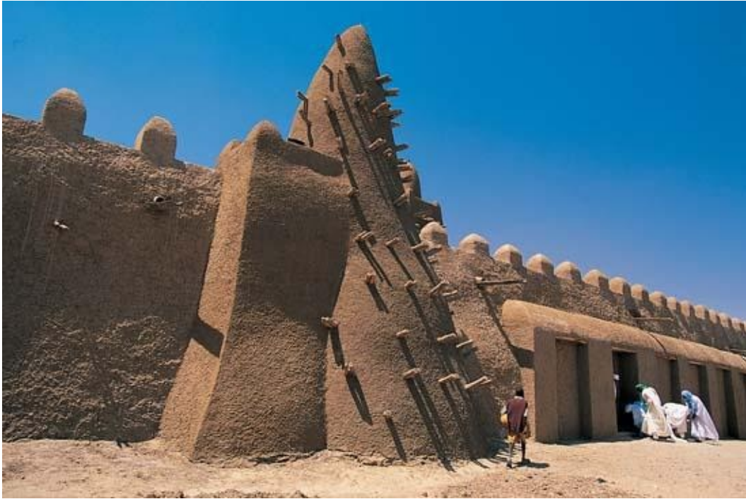
The newly restored walls of the 680-year-old Djingareiber Mosque in Timbuktu - the oldest mosque in continuous use in West Africa. It was built by El Saheli, the man credited with inventing this style of mud-brick architecture.
