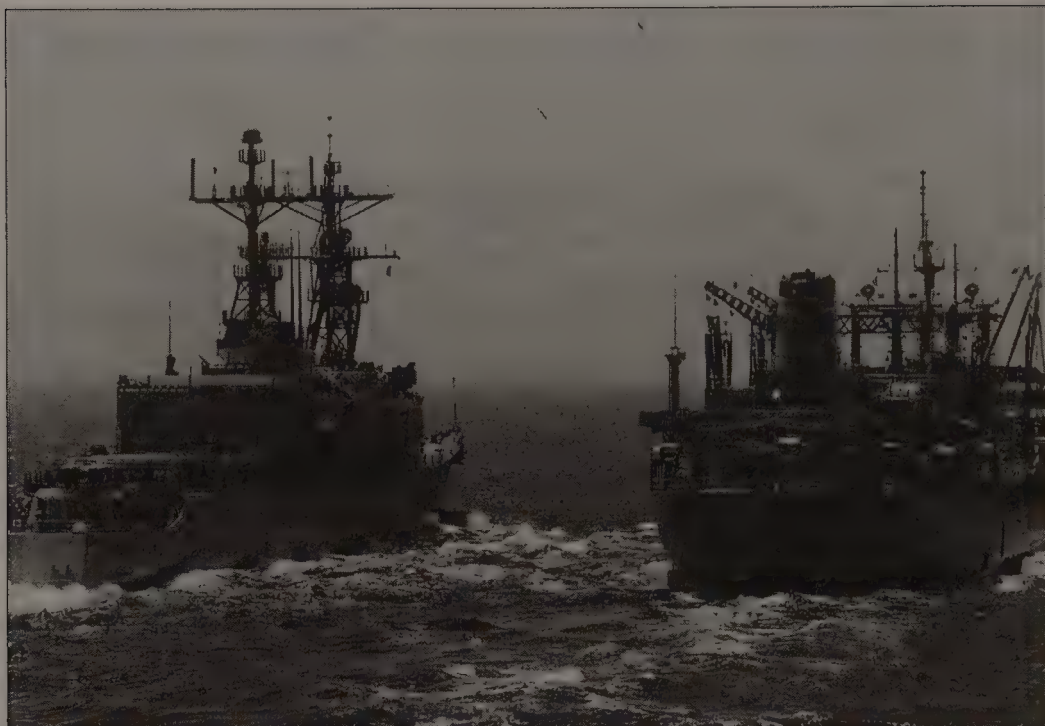
Figure 19.16. Underway replenishment (UNREP) allows ships to remain on station for long periods of time.
