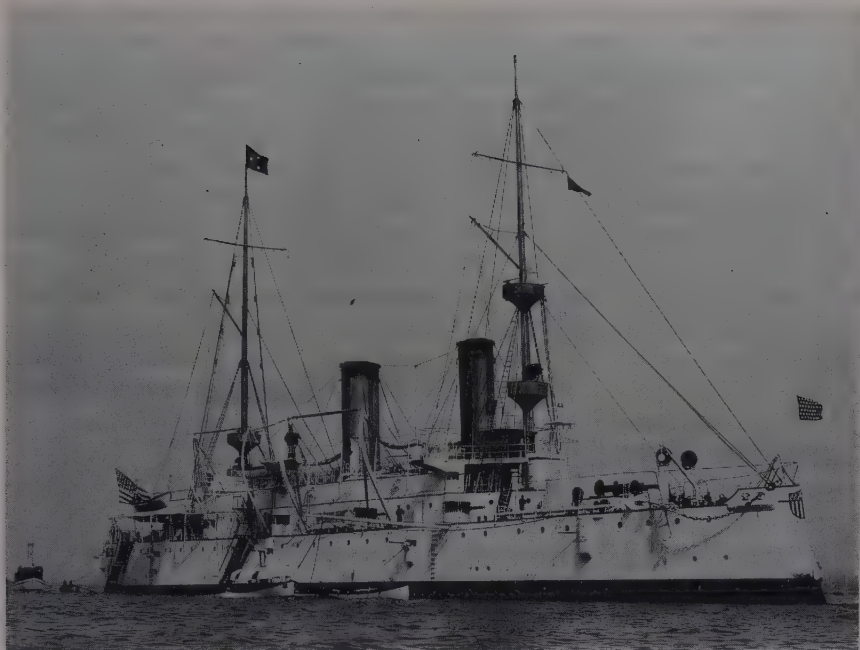
11. The USS Olympia in 1899, with Dewey's pennant at the main. "Protected cruisers" such as this were unarmored except for a deck at the waterline to shield their interiors from plunging fire. Commissioned in 1895, the Olympia displaced 5,586 tons, carried a crew of 411, and had a speed of 20 knots. Her main battery consisted of four 8-inch guns. Today she is preserved at Philadelphia, Pennsylvania. (Library of Congress photograph, U.S. Naval Institute Photographic Collection.)
