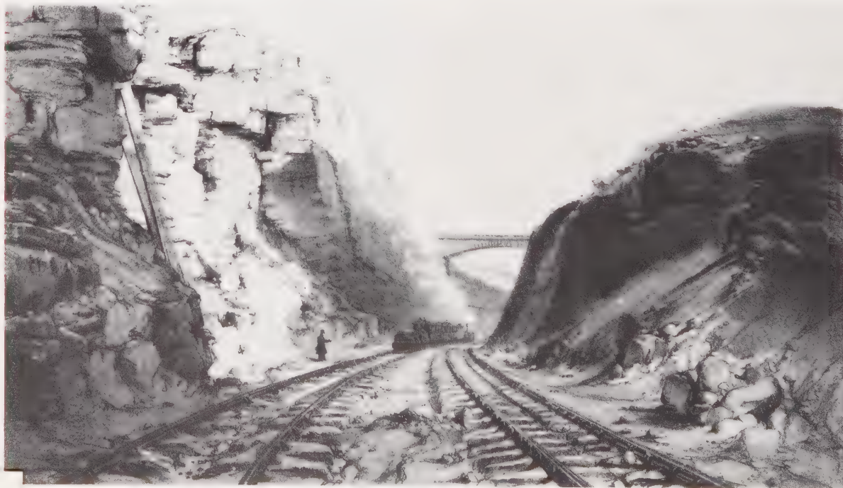
Plate 18: Blisworth cutting, London and Birmingham Railway. Note the stone sleepers.
