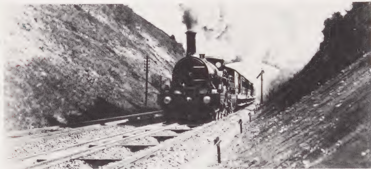
Plate 13: A broad gauge train on the Great Western Railway. The mixed gauge track allowed narrow gauge trains to work over the same line.
