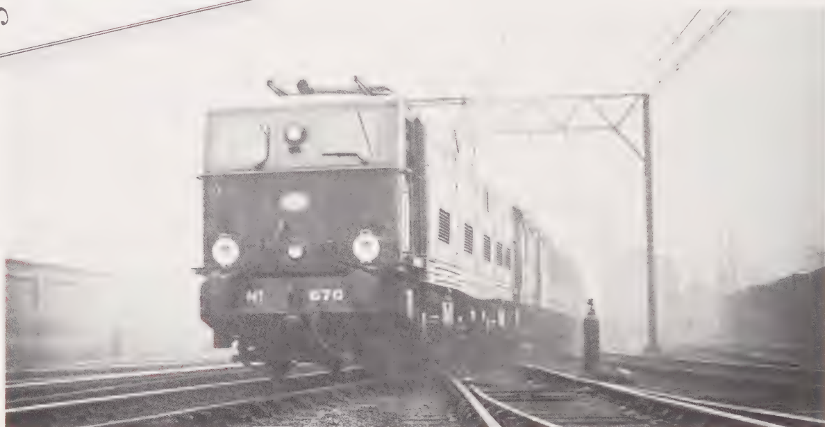
Plate 79: The LNER's late entry in the electrification stakes: the Manchester-Sheffield-Wath scheme. Here the prototype locomotive is seen on its trial run in October 1941.
