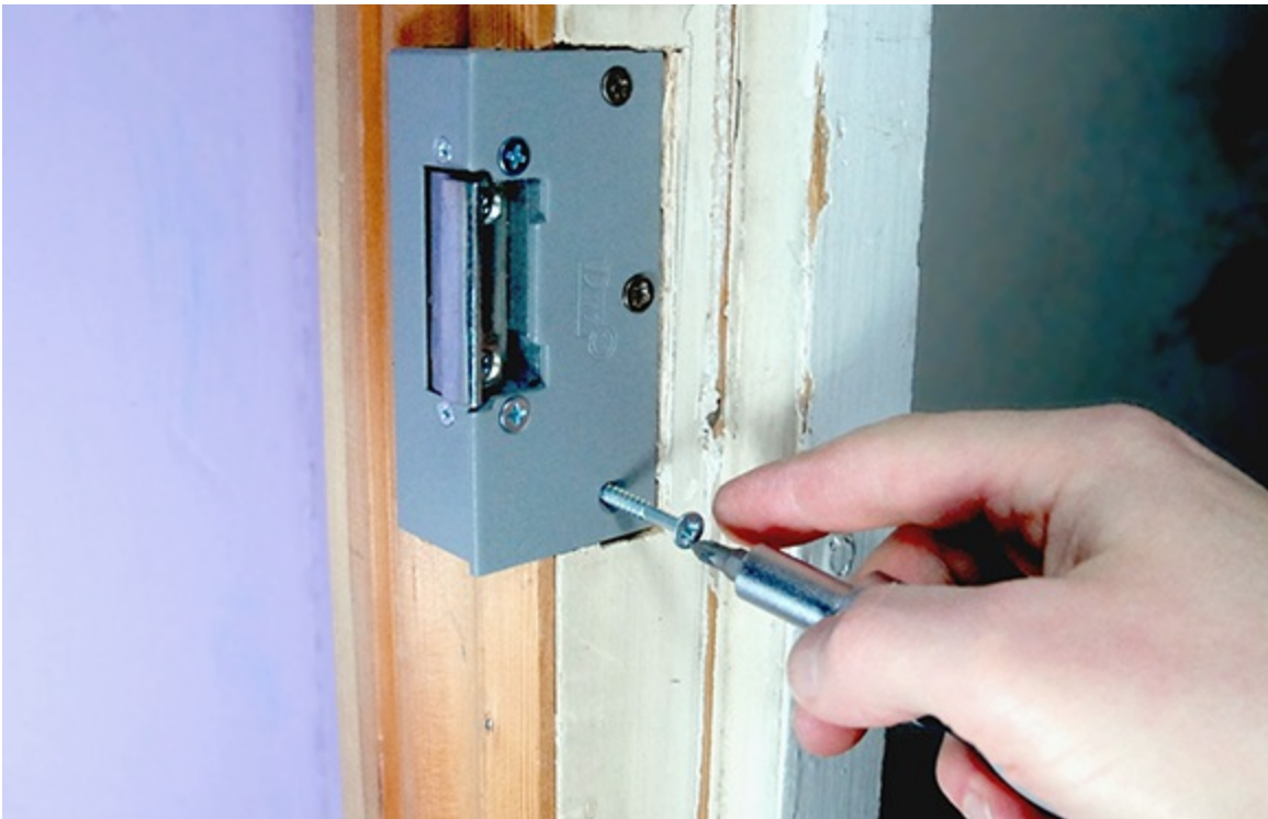
Figure 8-13: Installing the door strike.
