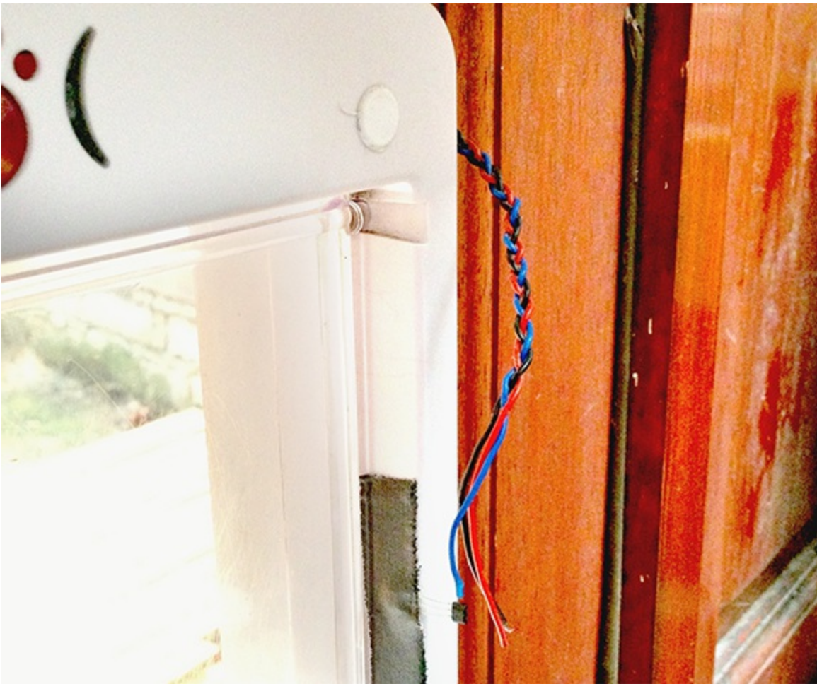
Figure 11-8: Taping your sensors in place to estimate the signaling wire length.
