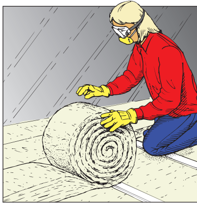
Figure 2-1: To add insulation to a loft, install poly-wrapped insulation at right-angles to existing insulation.
