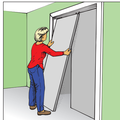
Removing a sliding door by lifting it up out of its tracks.
