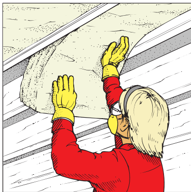
Figure 2-2: Pressing the insulation into cavities between the floor joists.
