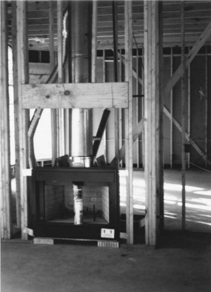
**Figure 10-2** Framed-in prefab fireplace sitting on bricks. Note the double exhaust pipe where once the house would have had a solid masonry construction. This type is primarily for decoration. However, it can be used for heat if necessary.
