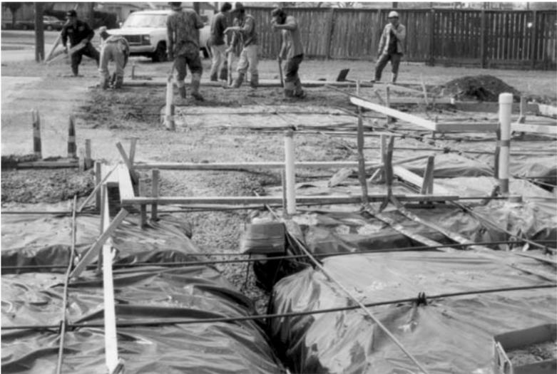
**Figure 2-15** Cables in place for the slab. Note trenching for plumbing and for footings and reinforcement for the slab. Site ready for concrete pouring.
