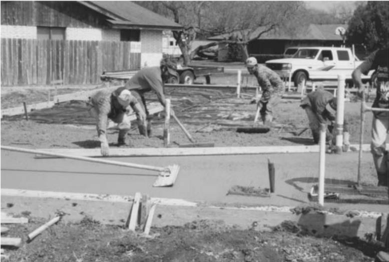
**Figure 2-16** Pouring the slab and leveling the concrete in the forms.
