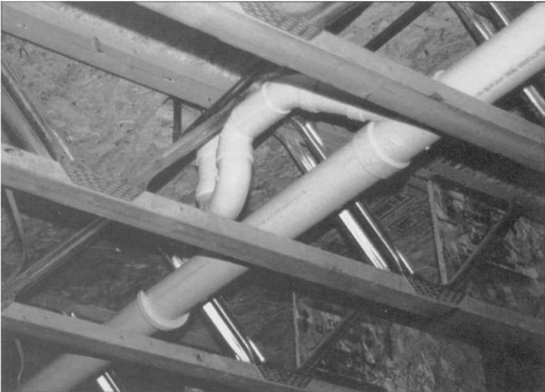
**Figure 8-8 Plumbing routed through the metal web of the joist.** (Courtesy of Truswal Systems Corp.)
