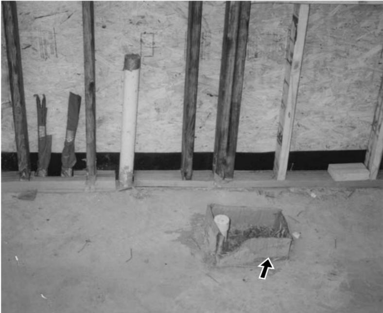
**Figure 3-13** Cardboard box being used as a form in a concrete floor-slab pour.
