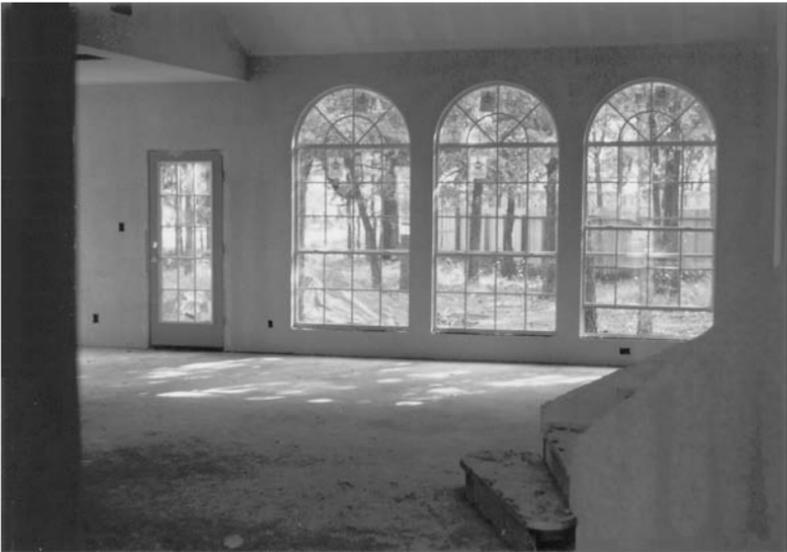
**Figure 15-7** Double-hung windows capped off with semicircular stationary “half-moons.”
