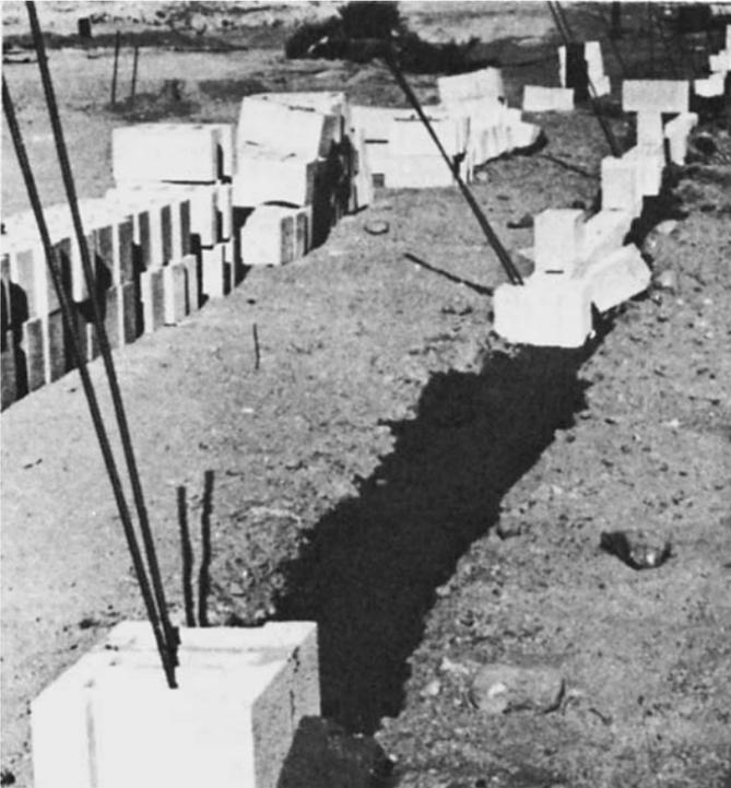
**Figure 5-14** Vertical reinforcement rods through double-thick column blocks.
