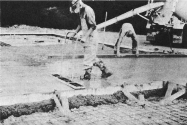
**Figure 2-6 Hand tamping, or jitterbugging, concrete to place large aggregate below the surface. The other worker (bent over) is screeding with a long  $2 \times 4$  to proper grade.**
