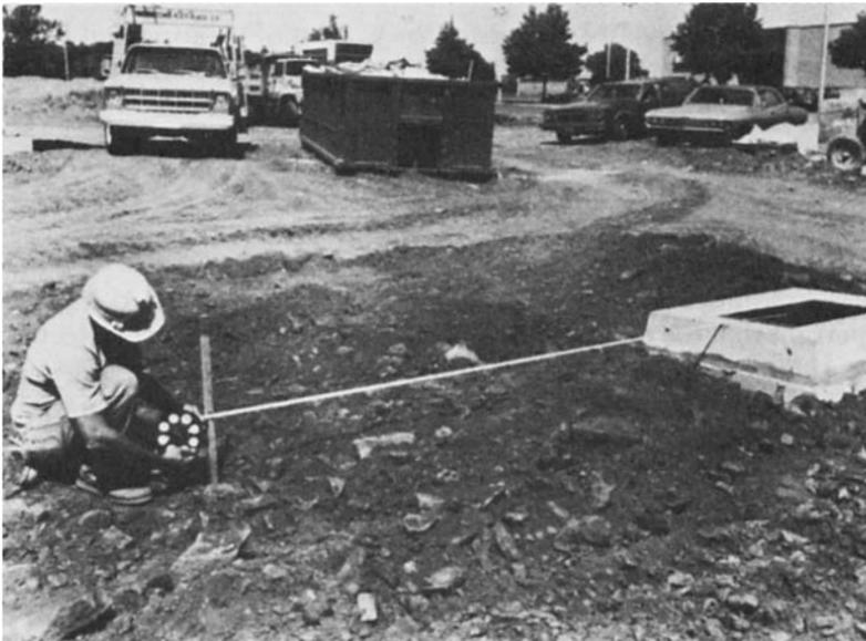
**Figure 1-1** One way of laying out is with a hundred-foot tape. Metal tape is standard, but this new fiberglass one works well and cleans easily. (Courtesy of Stanley Tools.)
