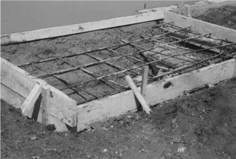
**Figure 2-17** Concrete slab poured. Rebar for porch ready for concrete.
