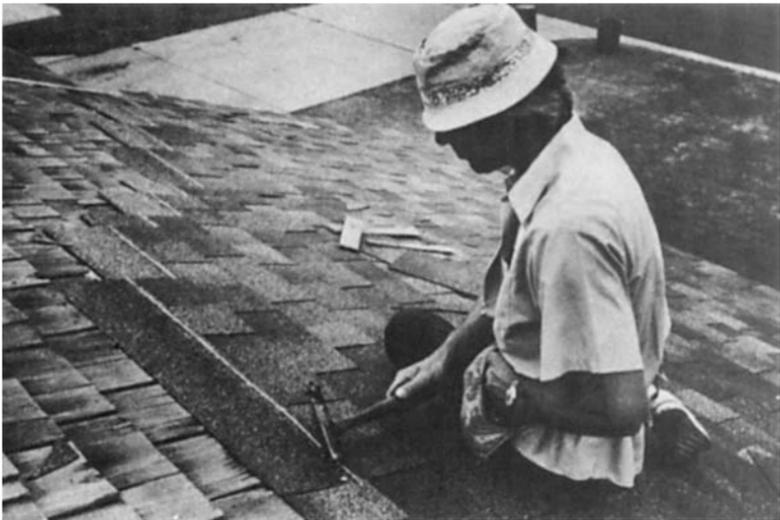
**Figure 11-2** Asphalt shingles being installed on a wood-shingle roof. Asphalt is now the most popular roofing.
