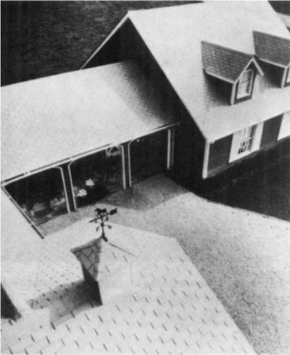
**Figure I I-3** Glass-fiber shingles are light in weight and have a high fire-resistance rating. *(Courtesy of Owens-Corning)*
