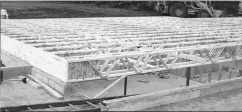
**Figure 8-11 Crawl-space construction on a slab with Space-Joist TE joists in place.** (Courtesy of Truswal Systems Corp.)
