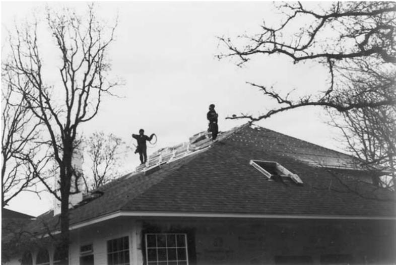
**Figure 11-19** Roofers pulling up their air hose to continue upward in the application of shingles.
