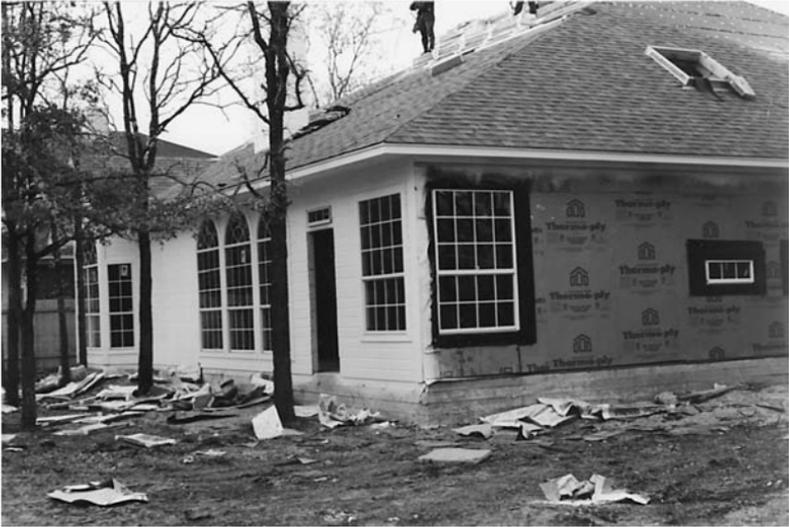
**Figure 11-20** Shingle wrappings create a safety hazard and become unsightly.
