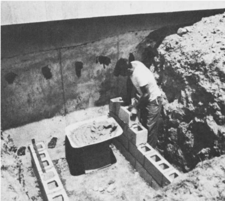
**Figure 5-1** Two-core masonry block being installed. (Courtesy of Bilco Company.)
