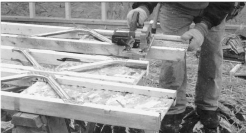
**Figure 8-9** Using a power handsaw to cut joist ends to fit. (Courtesy of Truswal Systems Corp.)
