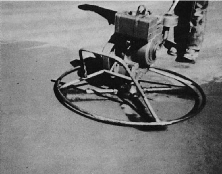
**Figure 2-9 Using a power trowel.**
