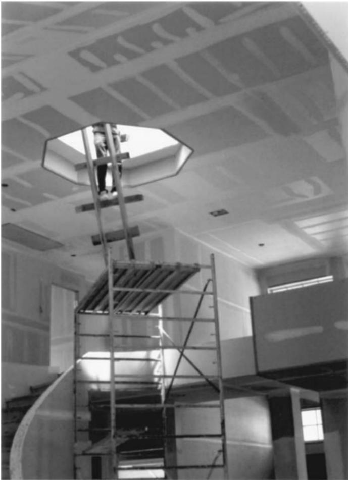
**Figure 12-5** Skylight viewed from inside during house construction.
