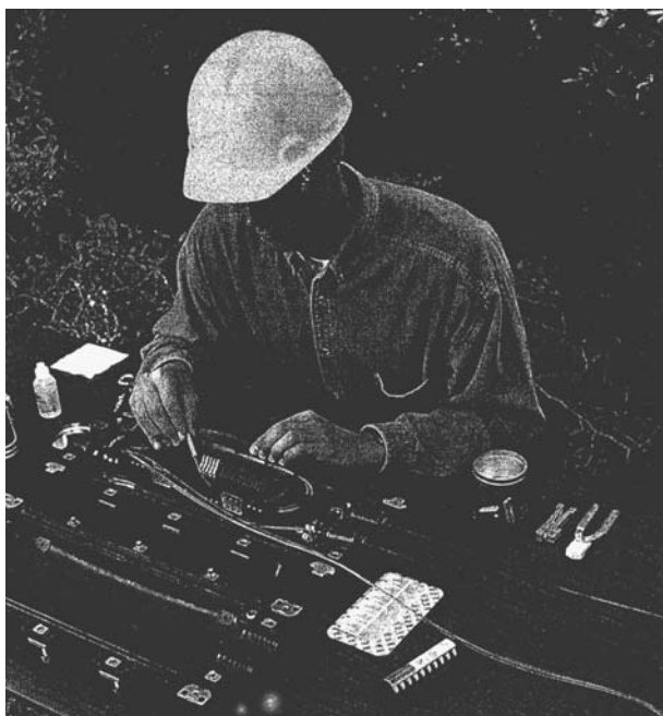
FIGURE 4.9 Craftsman populating an aerial closure with mechanical splices. (Fiber cleaver at right, bottle of index-matching gel at left.) [3M]
