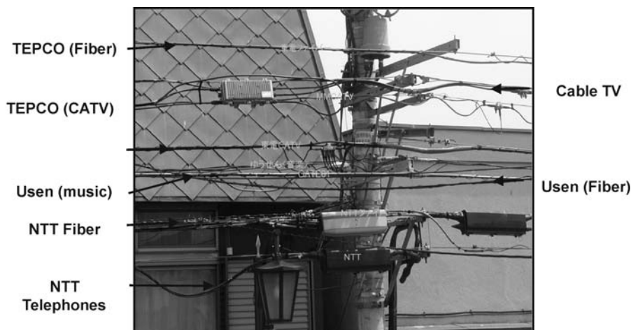
FIGURE 4.3 Street scene in a Tokyo residential area, illustrating the potential improvement to the visual environment promised by use of fiber's bandwidth for carrying multiple services.
