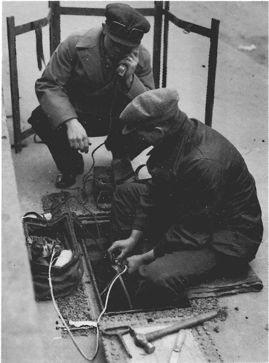
Figure 33.22 Streetside joint repair. Checking a joint during the installation of telephone service in 1935. Phoning the exchange. (Courtesy of BT Archives)
