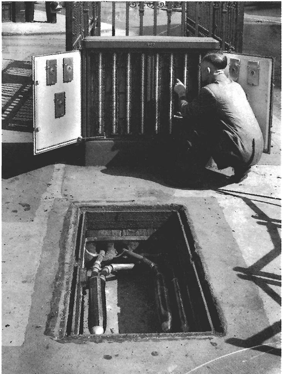
Figure 33.21 Streetside cabinet and jointing box. An engineer checking the wiring on the cross-connection frame inside a streetside cabinet. This provides for flexible connection of the many cables and individual pairs out to customers' premises and back to the exchange. In the foreground, the cables running away into the street conduits via a jointing box. ( Courtesy of BT Archives )
