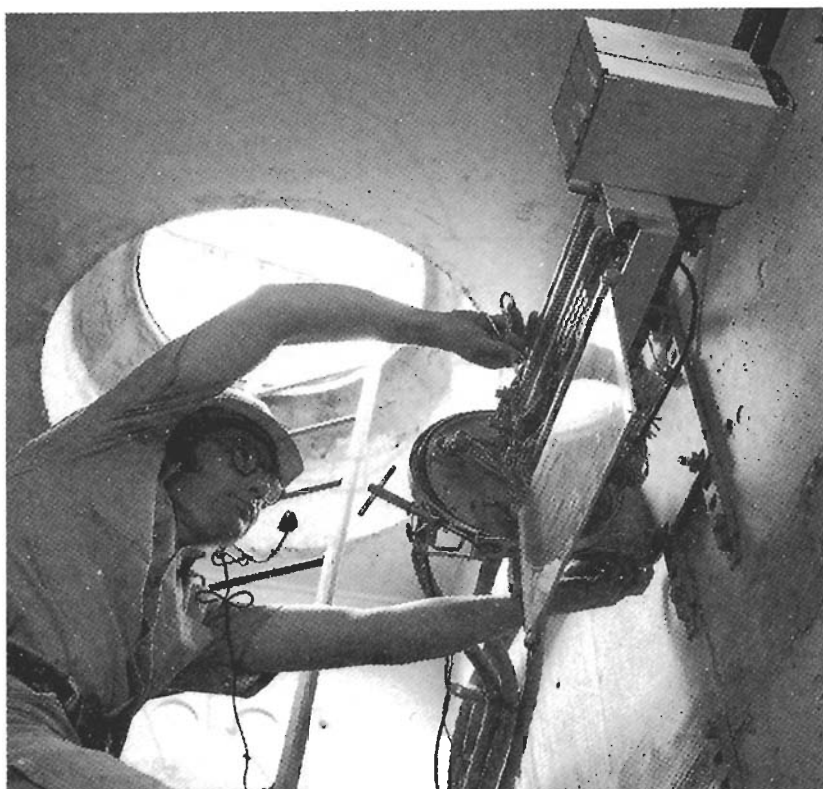
Figure 33.23 Metropolitan transmission system. In a sunlit manhole in New Jersey, USA, an installer checks out the wiring in a maintenance case – part of the Bell System's metropolitan transmission system. (Courtesy of AT&T)
