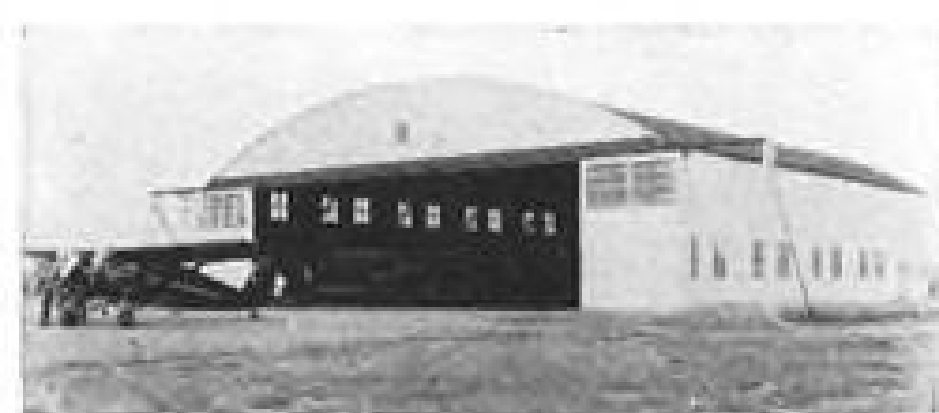
MUNICIPAL HANGAR. Timber Structures, Inc. supplied 5-80' trusses for this 80'x80' hangar. Architect: Victor E. Siebert. Contractor: O. D. Keen.
