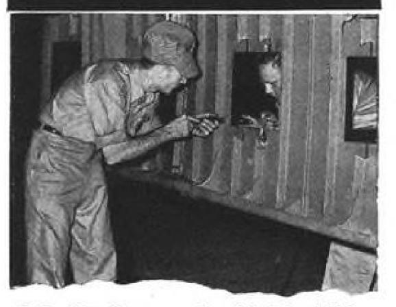
Reflecting floors made with Atlas White cement would materially increase illumination on this vertical work surface.
