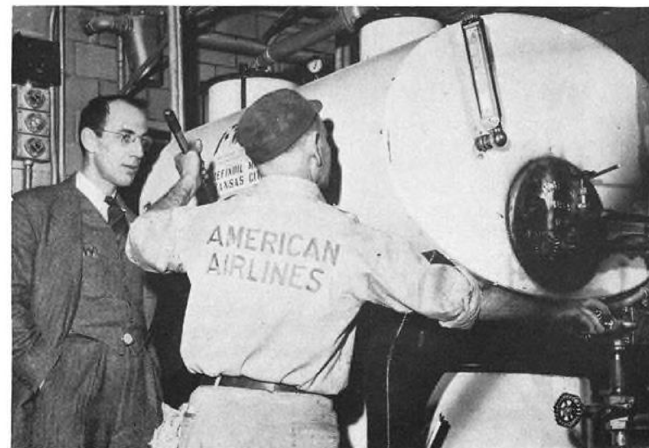
Airline Operates Oil Re-Refinery: American Airlines reports approximately 25 percent of the oil it uses is re-refined lubricating oil. Here Gilbert K. Brower, materials engineer and director of the program, watches a worker make an adjustment at a re-refining machine at New York.
