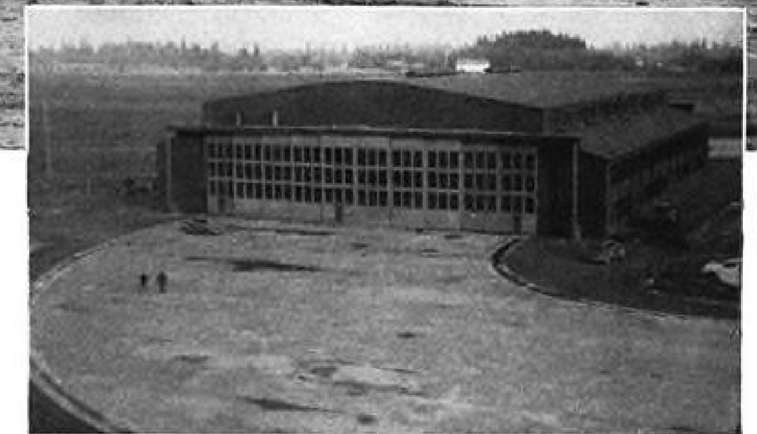
THIRTEEN 122' GLUED LAMINATED TRUSSES, columns, purlins, framing, hangar doors supplied by Timber Structures, Inc.
