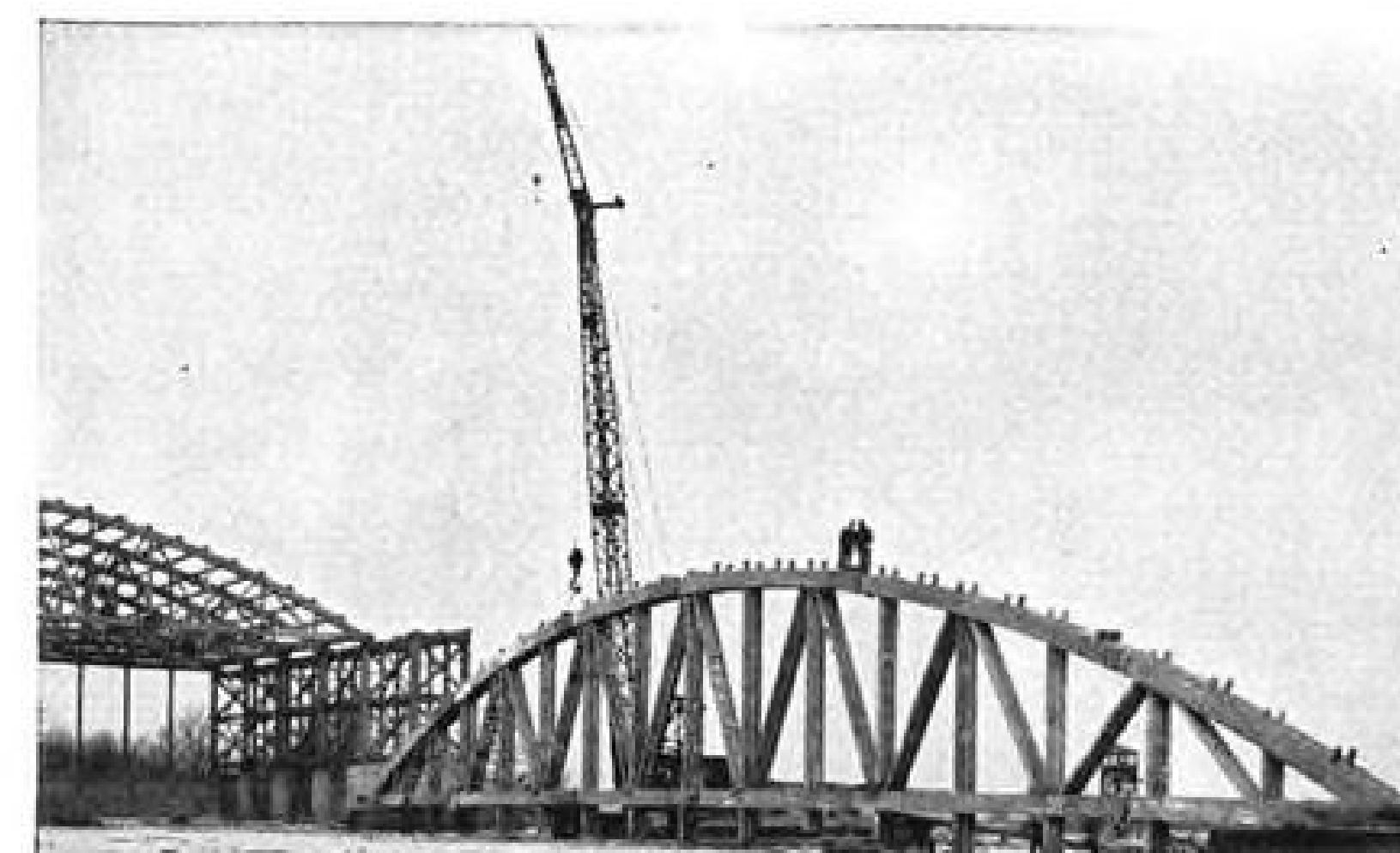
LARGEST of their kind are the 12-200' laminated trusses for this aircraft plant. Center chords of the front trusses are built up of 1 3/4"x5 1/2" lumber; 14 laminations in the lower chord; 15 laminations in the upper chord. Intermediate truss chords are built up of 1 3/4"x3 5/8" lumber; 13 laminae in lower chords; 14 laminae in upper chords. Timber Structures is now building similar trusses for another project, this time using spans of 223' center to center of bearings.
