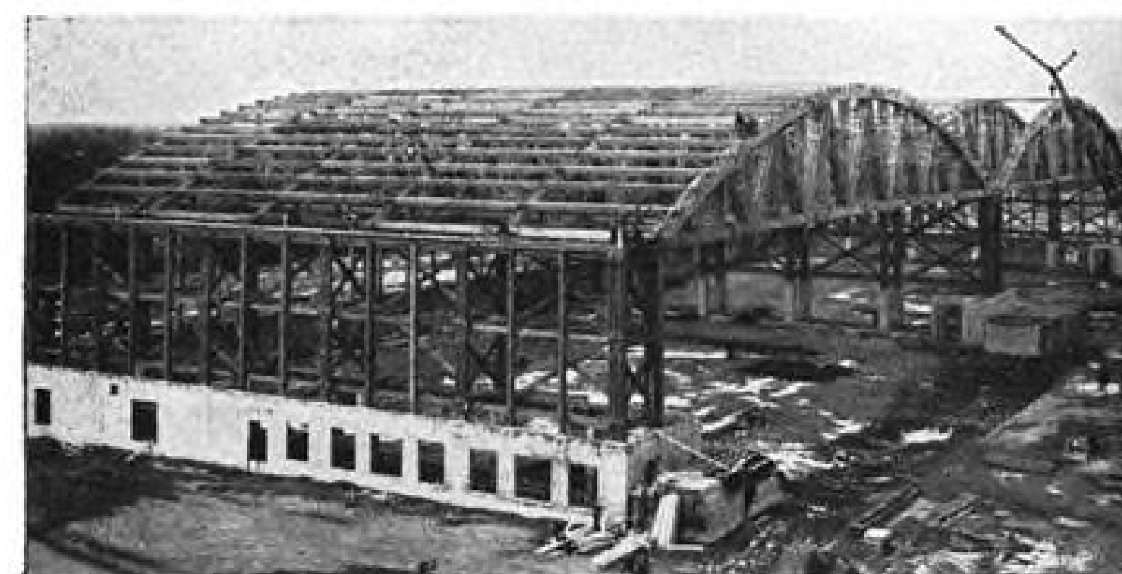
LARGEST of their kind are the 12-200' laminated trusses for this aircraft plant. Center chords of the front trusses are built up of 1 3/4"x5 1/2" lumber; 14 laminations in the lower chord; 15 laminations in the upper chord. Intermediate truss chords are built up of 1 3/4"x3 5/8" lumber; 13 laminae in lower chords; 14 laminae in upper chords. Timber Structures is now building similar trusses for another project, this time using spans of 223' center to center of bearings.
