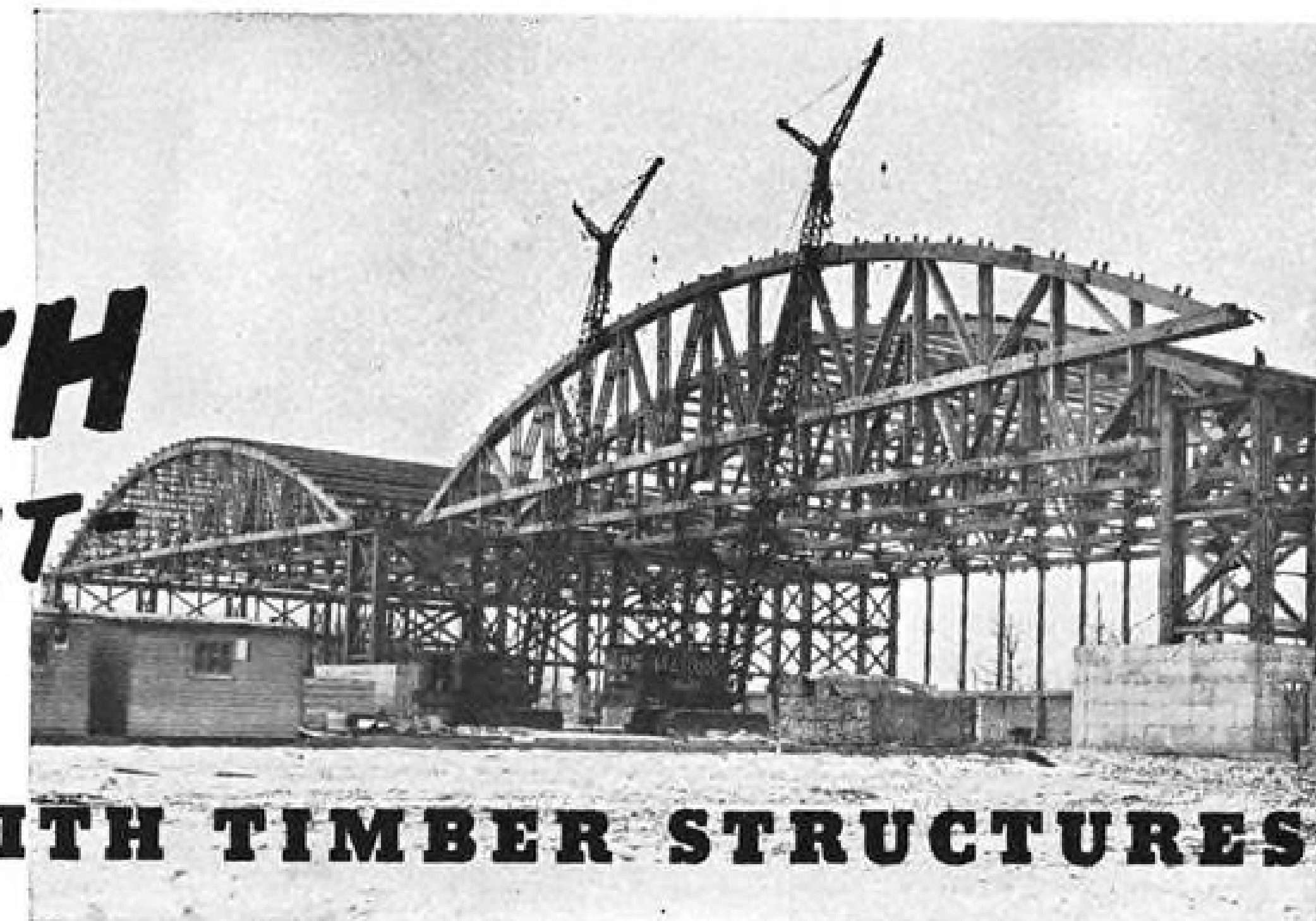
CLEVELAND. 200' laminated trusses were designed, prefabricated and erected by Timber Structures, Inc. for 200'x440' assembly plant, for The U.S. Engineers. Front trusses, (supporting doors and roof), were built to carry 450,000 lbs. Intermediate trusses built to carry 310,000 lbs.
