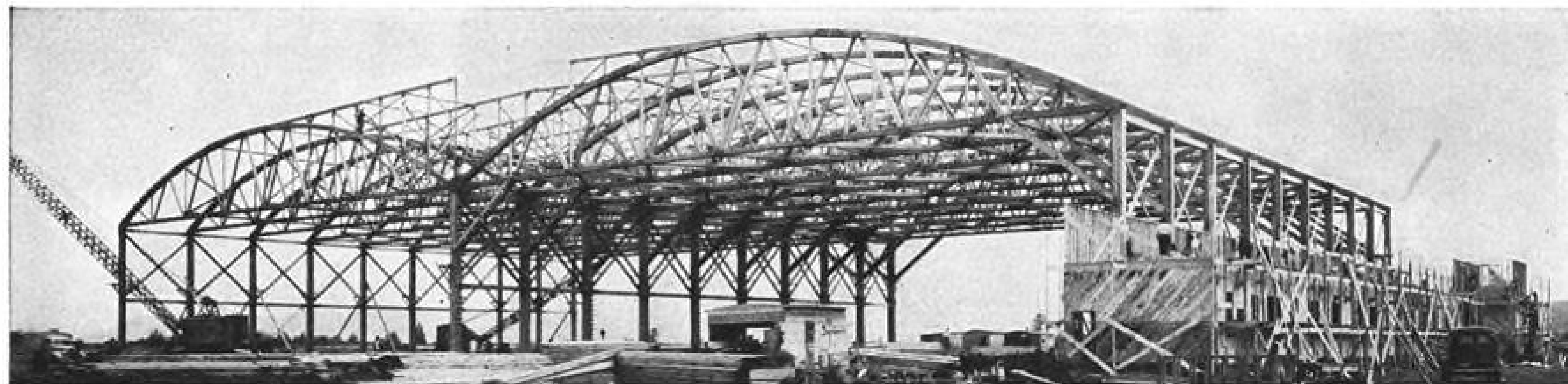
NAVY AIR BASE HANGAR (302'x180') Twenty 151' glued-laminated columns were fabricated for this two bay hangar by Timber Structures, Inc. Engineer and contractor: The Austin Company.
