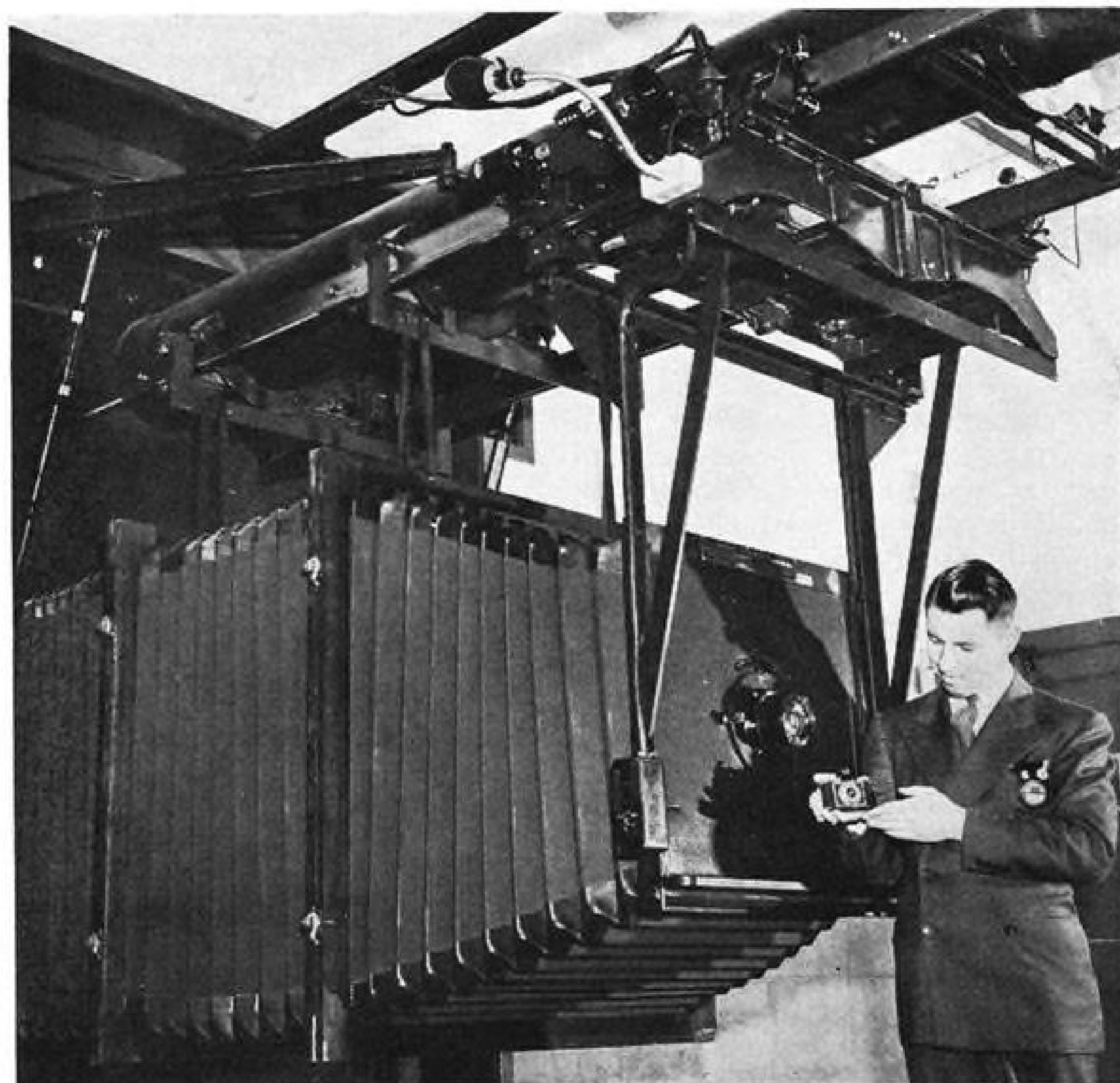
Boeing's Six Ton Camera: Glenn H. Jones, Boeing's photo template chief, contemplates a vest-pocket version beside the 12,000-pound model that speeds template work on Flying Fortresses .
