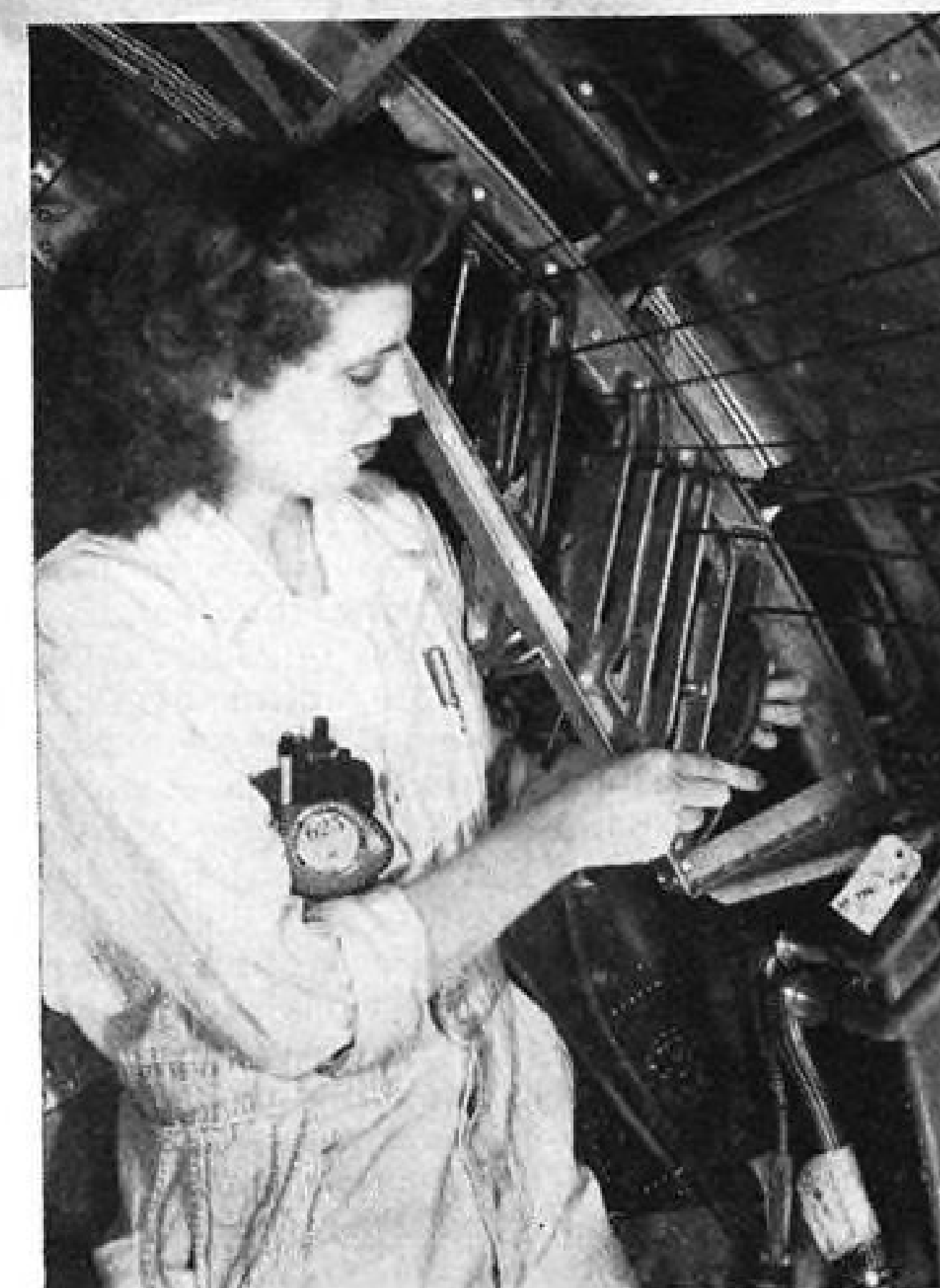
A bank of Fafnir equipped pulleys in the Boeing B-29 Superfortress
