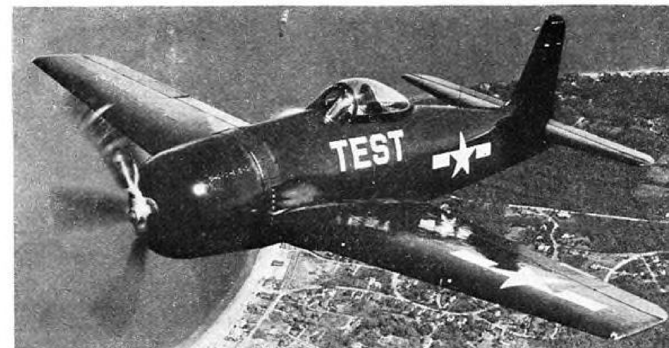
New Views of F8F “Bearcat”: This lightweight, high powered fighter, built by Grumman for the Navy, is smaller than its close kin, the Hellcat and Wildcat. Consequent lower drag makes it possible to put more aboard carriers, and the high horsepower makes it possible for them to take off with almost zero wind coming over the flight deck. The nearly 20 knot wind needed by most shipboard fighters has been a handicap to escort carriers.
