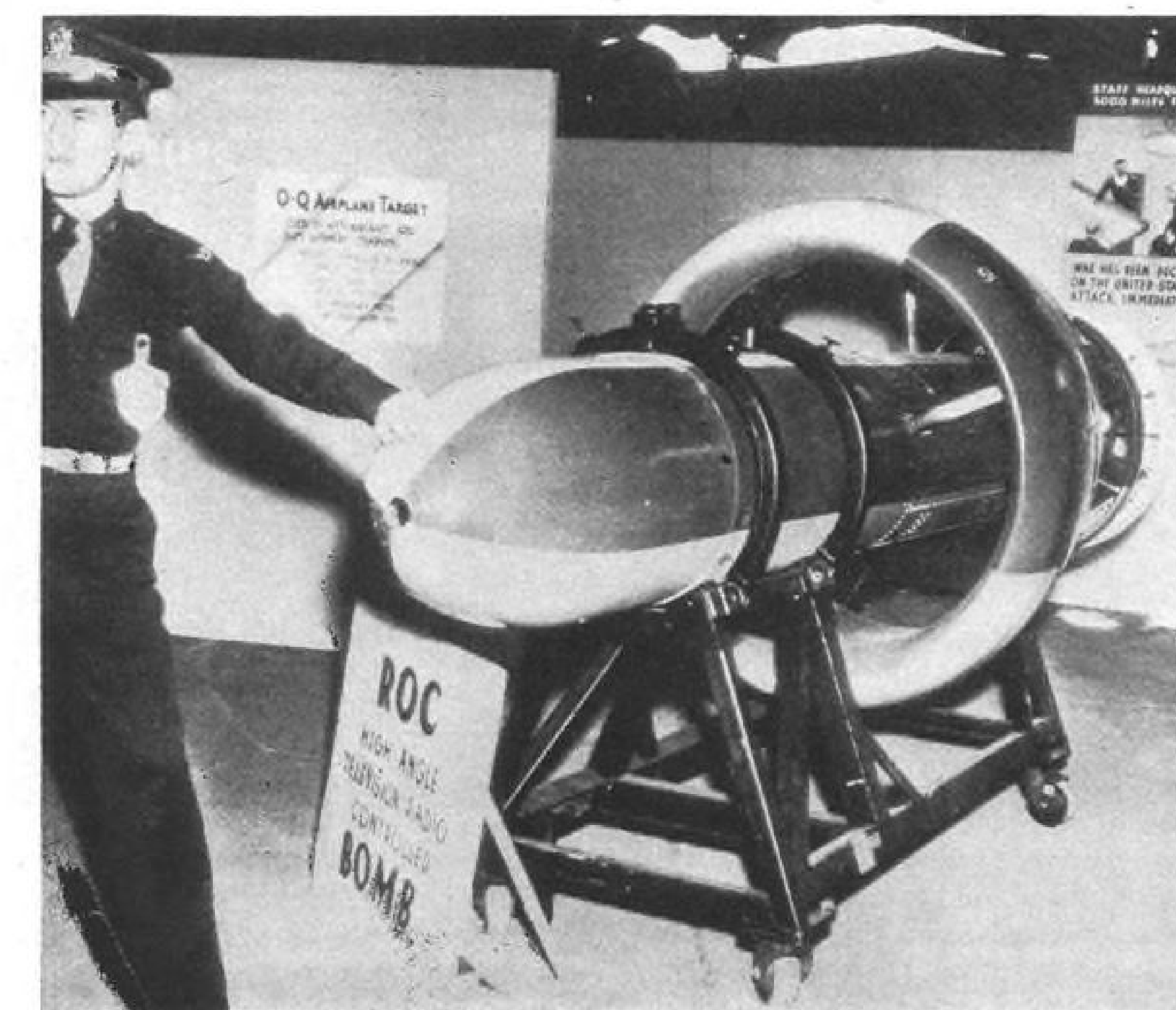
Television Bombs: Two versions of television-radio-controlled bombs, were unveiled for the public last week at the Air Fair held by Air Technical Service Command at Wright Field, Ohio. The GB-4 glider bomb, above, and the ROC high-angle bomb, below, both have television transmitters in their noses which send a continuous picture of where they are heading. The image is flashed on a screen in the plane from which they have dropped, so that the bombardier, by manipulating radio controls, can correct their fall if necessary, putting them "on target."
