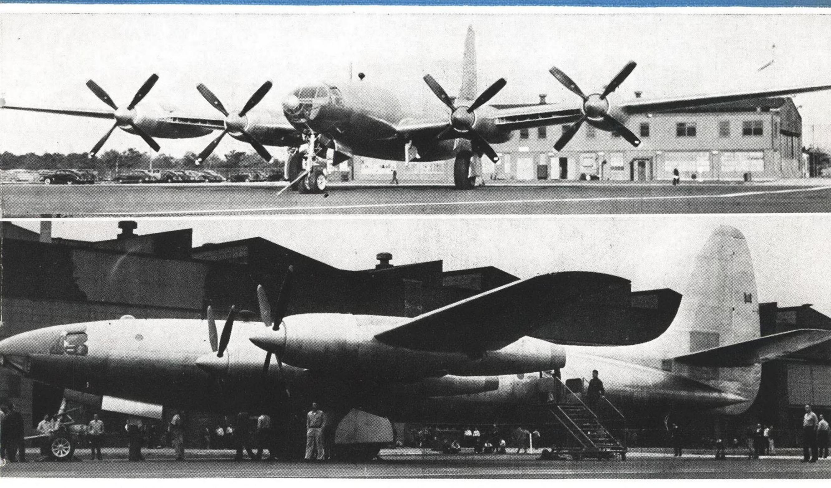
New Republic Giant: This XF-12, huge high-speed, long-range photo reconnaissance plane, was unveiled today at the Republic plant in Farmingdale, N. Y. With a span of 129 ft. 2 in. and a length of 98 ft. 9 in. the XF-12 is powered by Pratt & Whitney Wasp Majors which have been equipped with turbo exhausts through which Republic engineers hope to recover up to one-third of original engine output. The firm's forthcoming Rainbow transport will be based on this ship. (Story on Page 10.)
