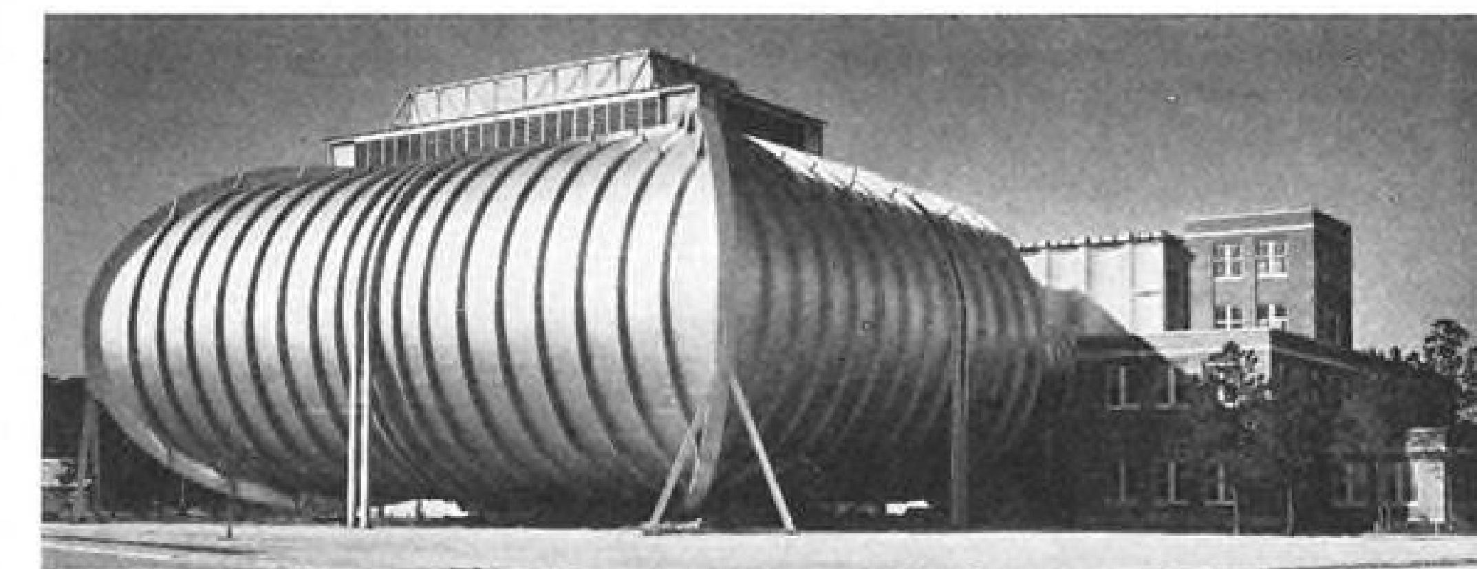
High-Speed Wind Tunnel: This 16-ft. high-speed wind tunnel at the Langley Field NACA laboratory is the scene of careful check-ups on flight characteristics of proposed planes.
