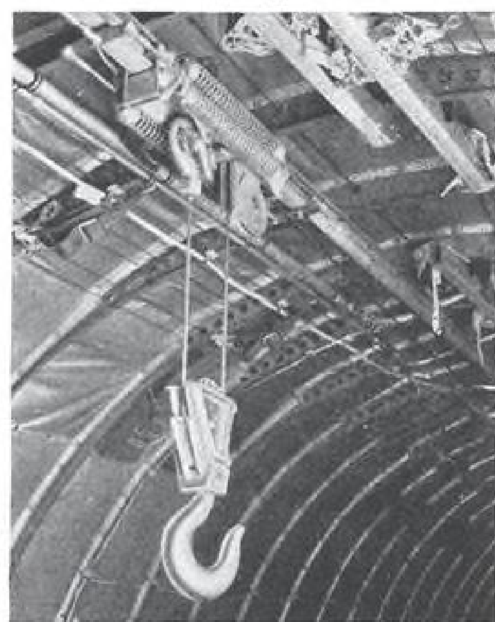
Powerful electric hoist on overhead rail facilitates loading of huge upper deck.
