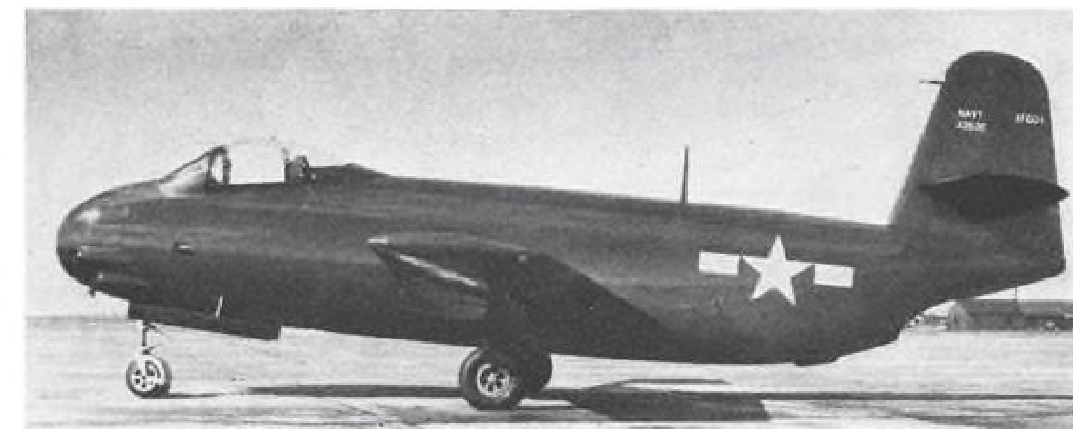
Successor to the Corsair: One of the latest additions to the Navy's rapidly growing stable of jet fighters is the Chance Vought XF6U-1. Built of a new type of material known as "Metalite" the Vought jet plane is powered by a new type Westinghouse jet. (Navy photo)
