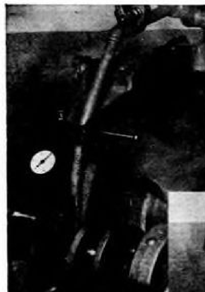
Gage rides on the work throughout the grinding operation.
