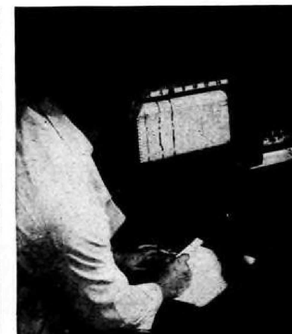
Electronic temperature recorder is used to determine completeness of combustion and to accurately record output temperatures.
