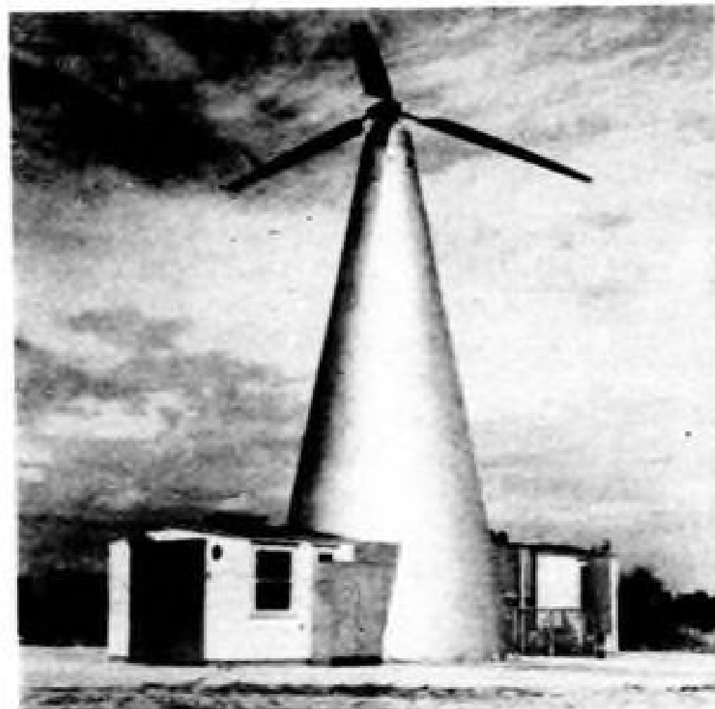
HELICOPTER WHIRL TEST TOWER —First photo of new 40 ft. NACA helicopter test tower at Langley Field, Va. shows three-blade Sikorsky R-6 rotor mounted on the tower for preliminary calibration tests of the tower. Motor-driven shaft will turn rotors as large as 60 ft. diameter. Tip speed problems, aerodynamics, flutter and vibration will be analyzed with the use of this new research facility. (Details on Page 21)
