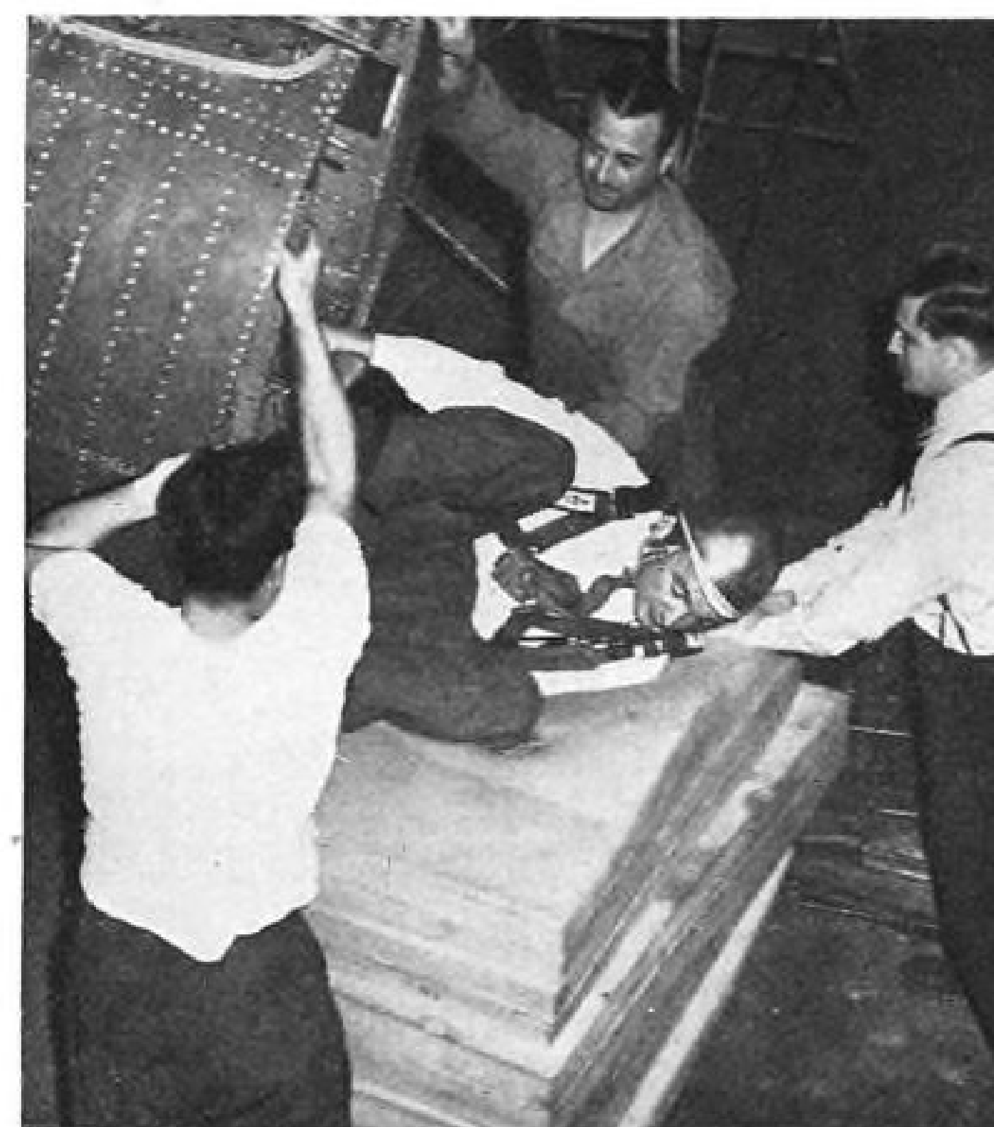
Photos show two methods of leaving nose section after emergency detachment. At left pilot rolls out. At right pilot backs from cockpit.
