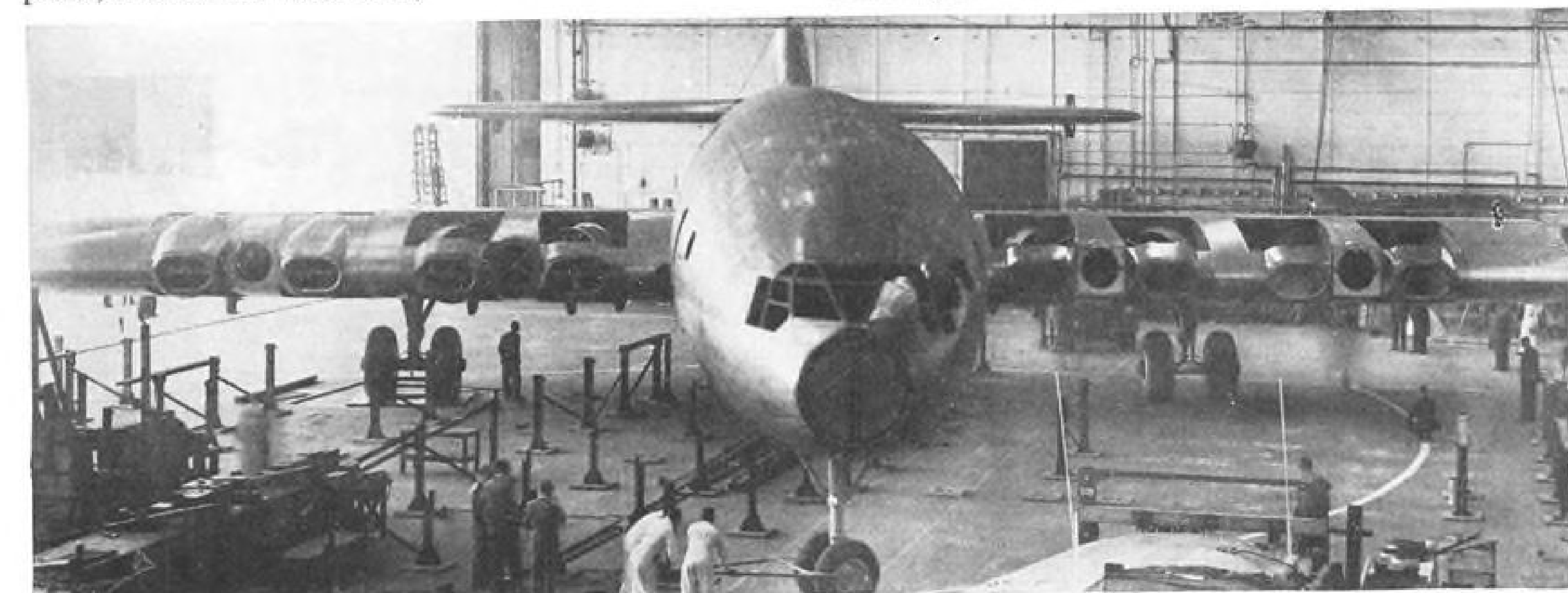
Front view clearly shows novel arrangement of engine nacelles. Each pair of engines will drive one contra rotating propeller.
