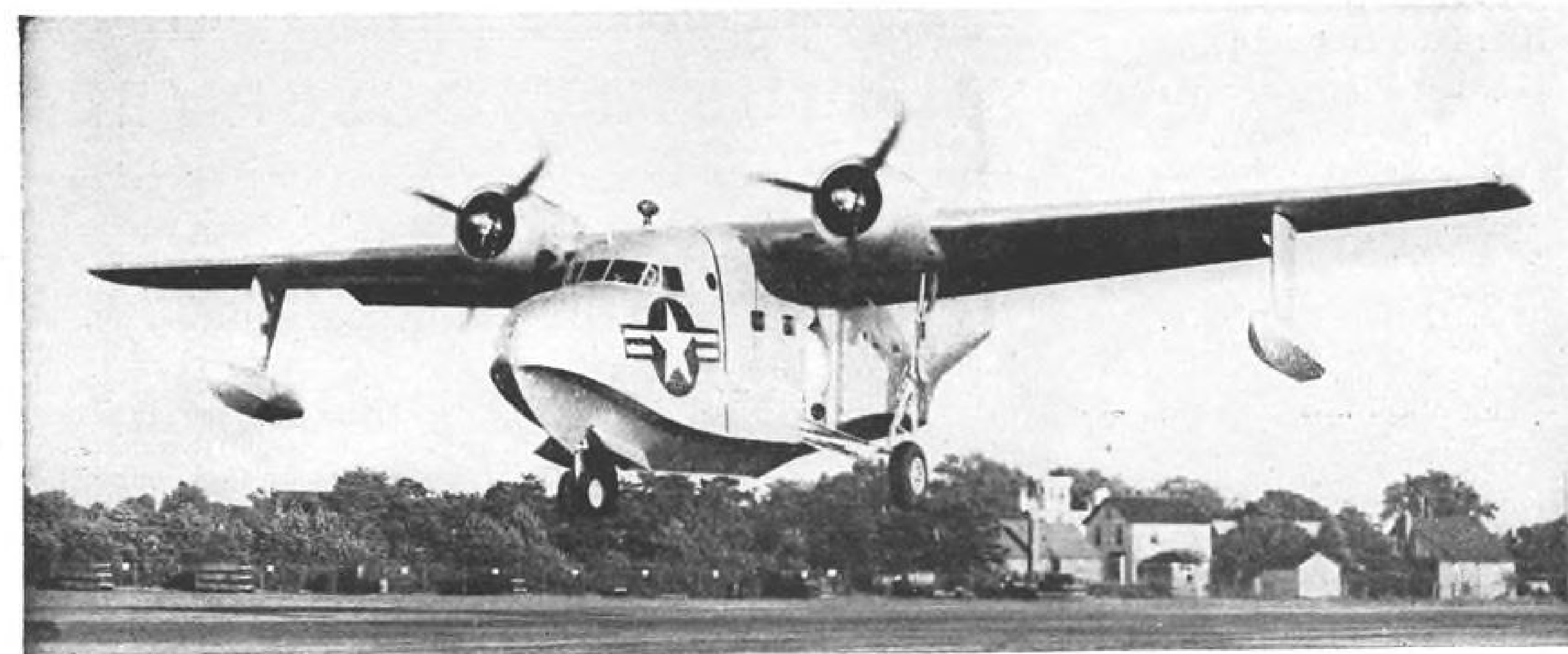
ENLARGED GRUMMAN MALLARD: First photo of Grumman XJR2F-1, enlarged version of the commercial Mallard, shows new Navy transport coming in to land after early test flight. Twin engine amphibian carries crew of three, 14 passengers or 16 litters as rescue plane. Cargo version can carry two tons. Big craft, as yet unnamed, cruises at 180 mph. Two have been ordered. (Navy photo)
