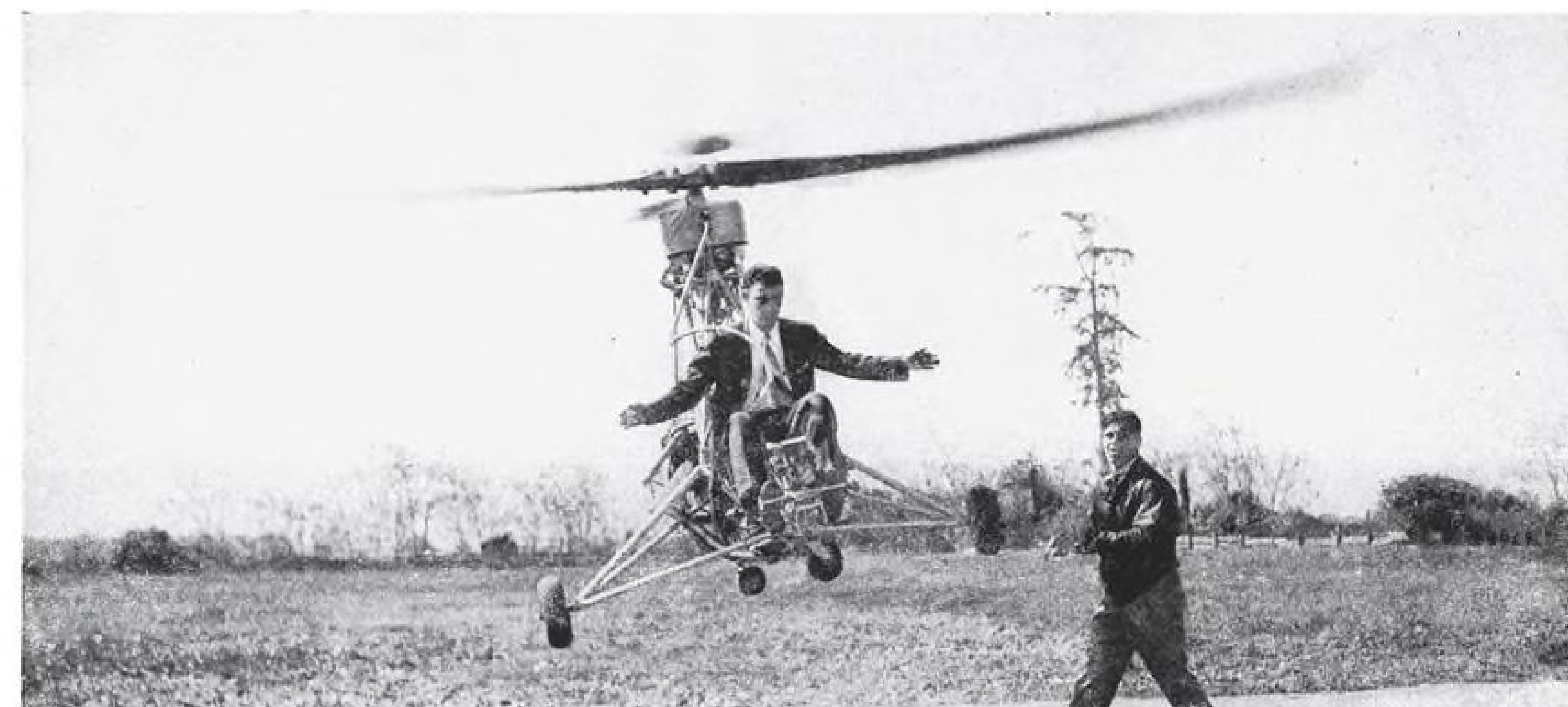
After ground aide has started helicopter swinging, it regains motionless hovering within three oscillations although pilots hands are off stick.
