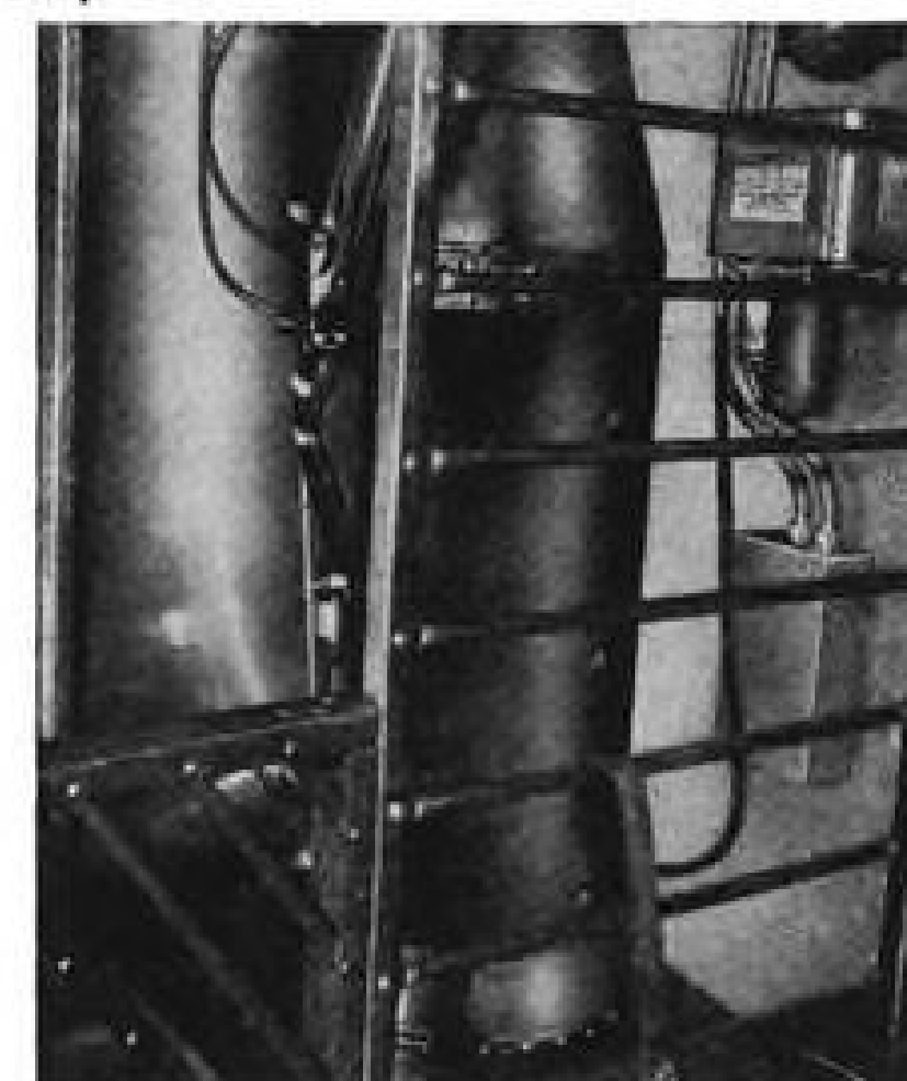
Note compactness and easy accessibility of heater and controls for inspection or servicing.
