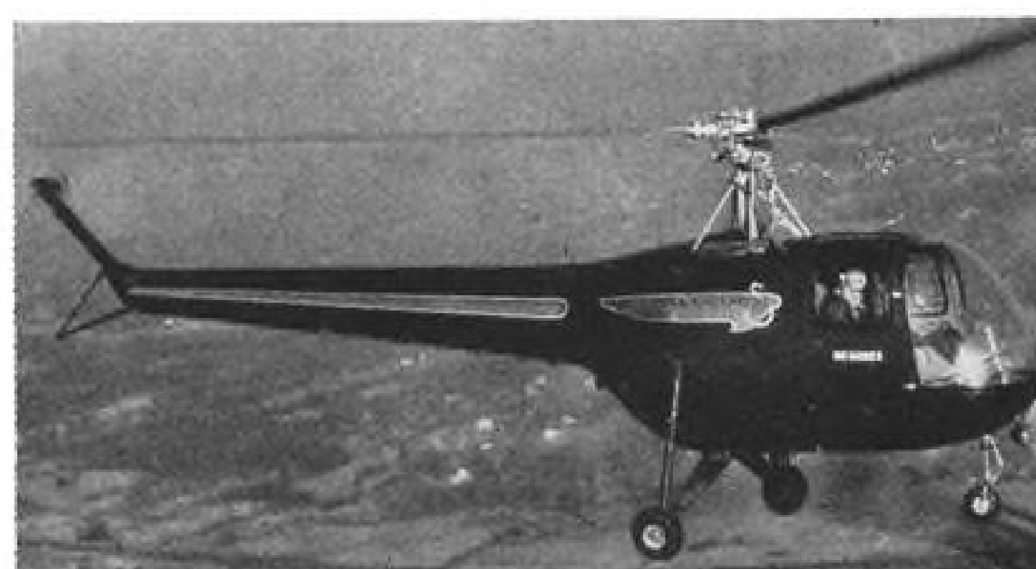
KAMAN K-125-A was designed as an engineering test stand for the development of their rotor systems.
