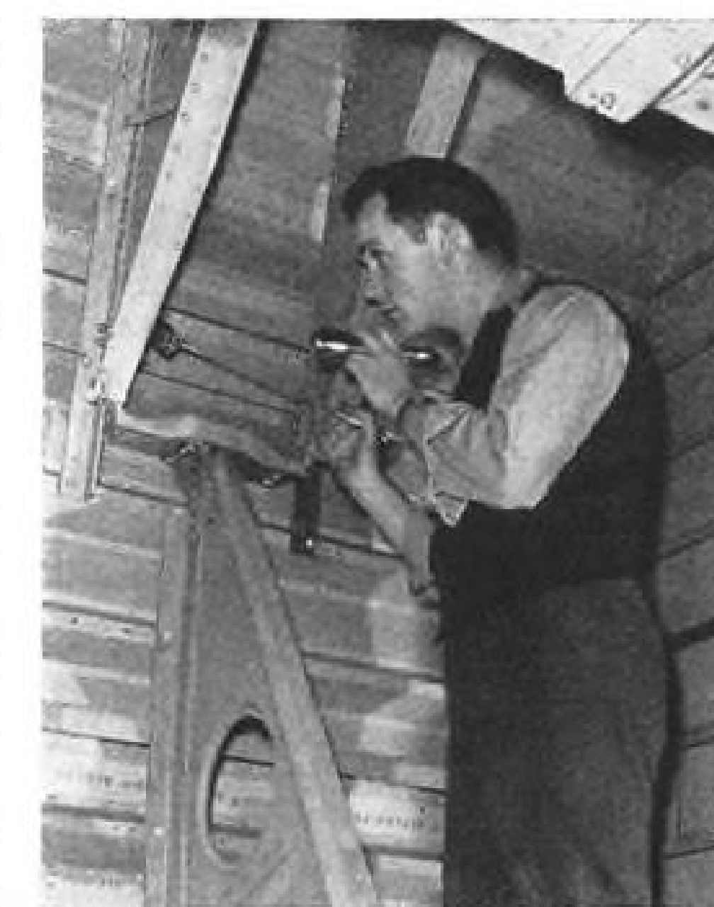
Inspector uses mirror and flashlight to check rivet formation in inaccessible location.
