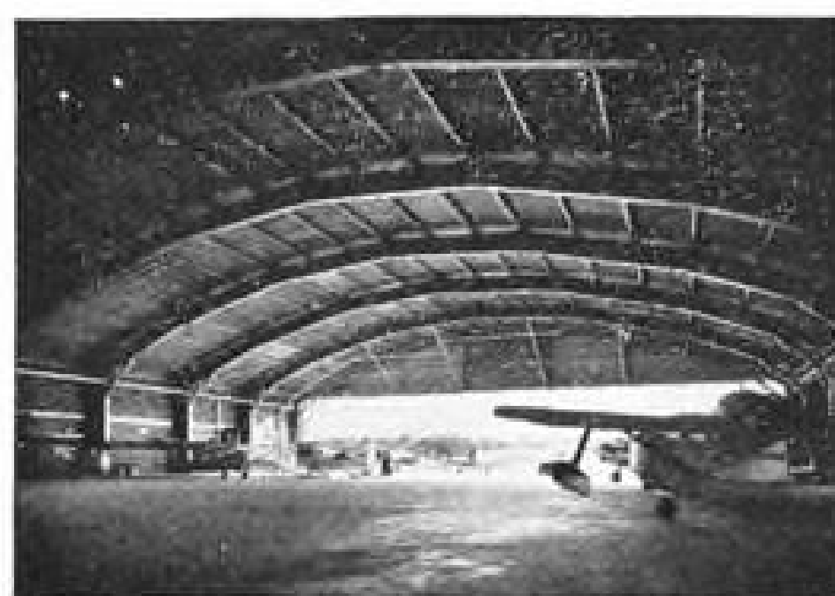
Interior view of Westchester hangar, showing girder-type roof construction.
