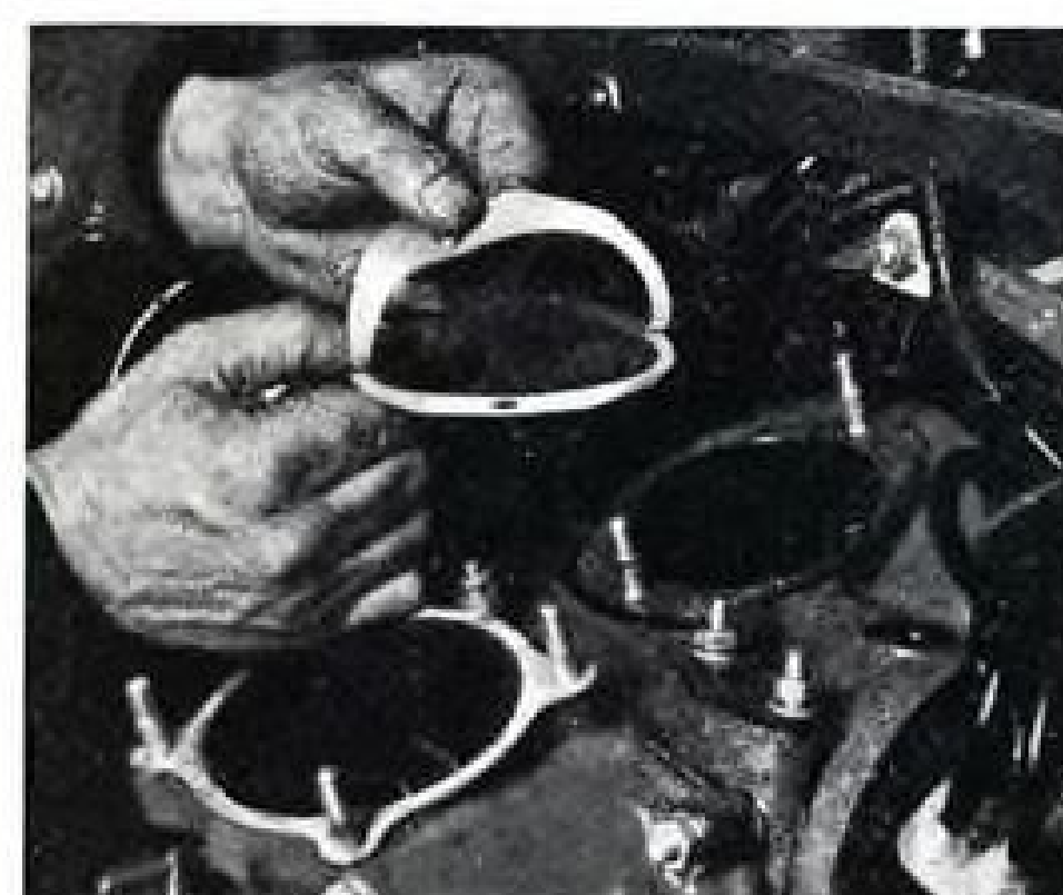
Using .002 inch laminations on magneto mounting and gear adjustment
