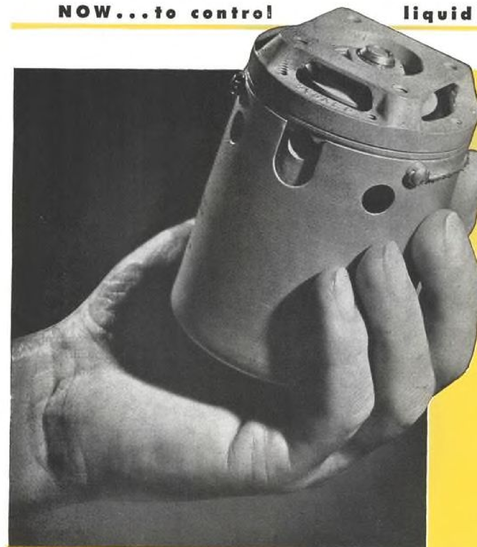
1 1/4" bottom-filling valve* as used on Republic F-84 Thunderjet.
