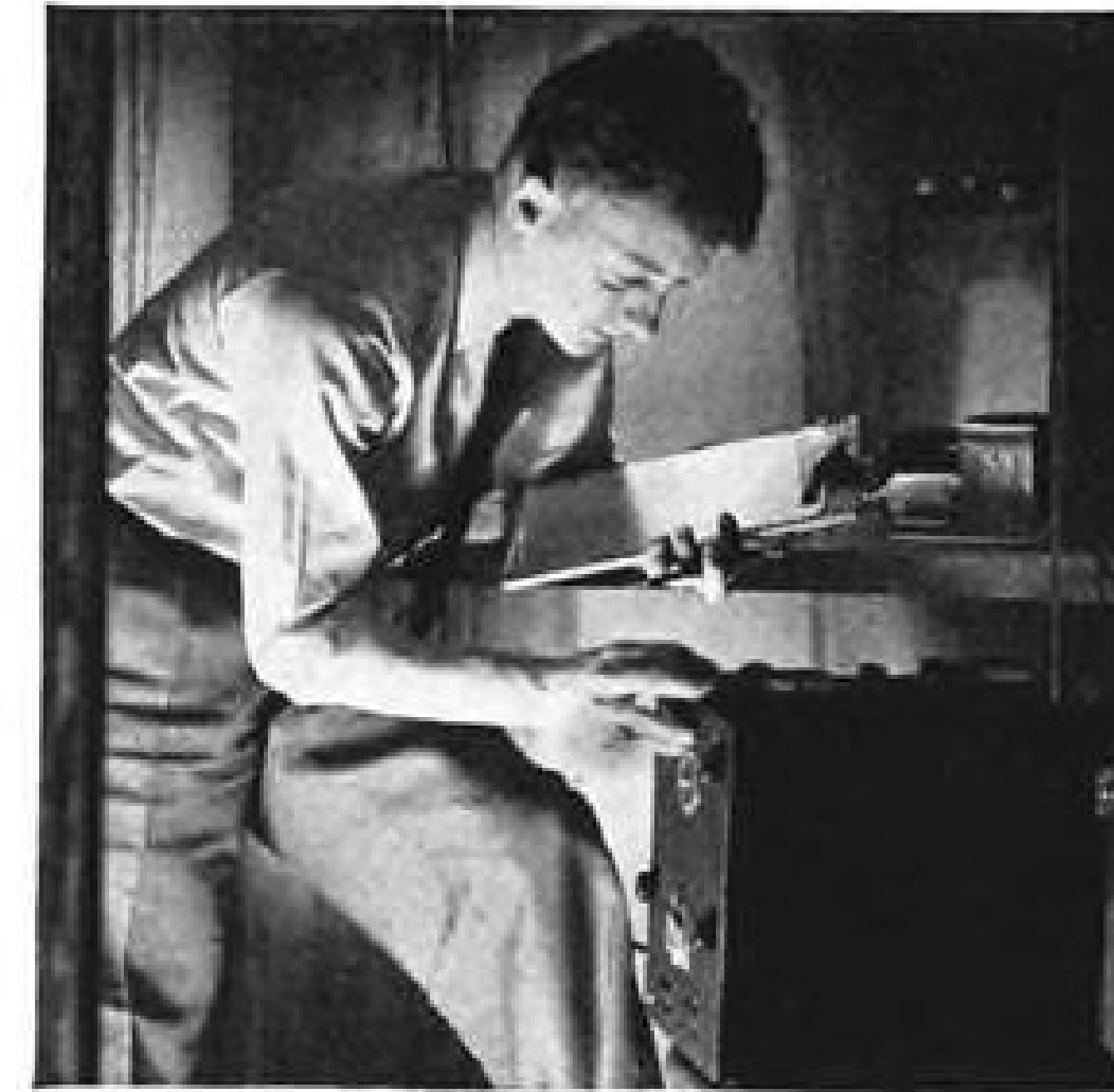
Quiet please. In this shielded "radio quiet" room, Janitrol electrical components are checked to insure against their producing unwanted interference with radio equipment.
