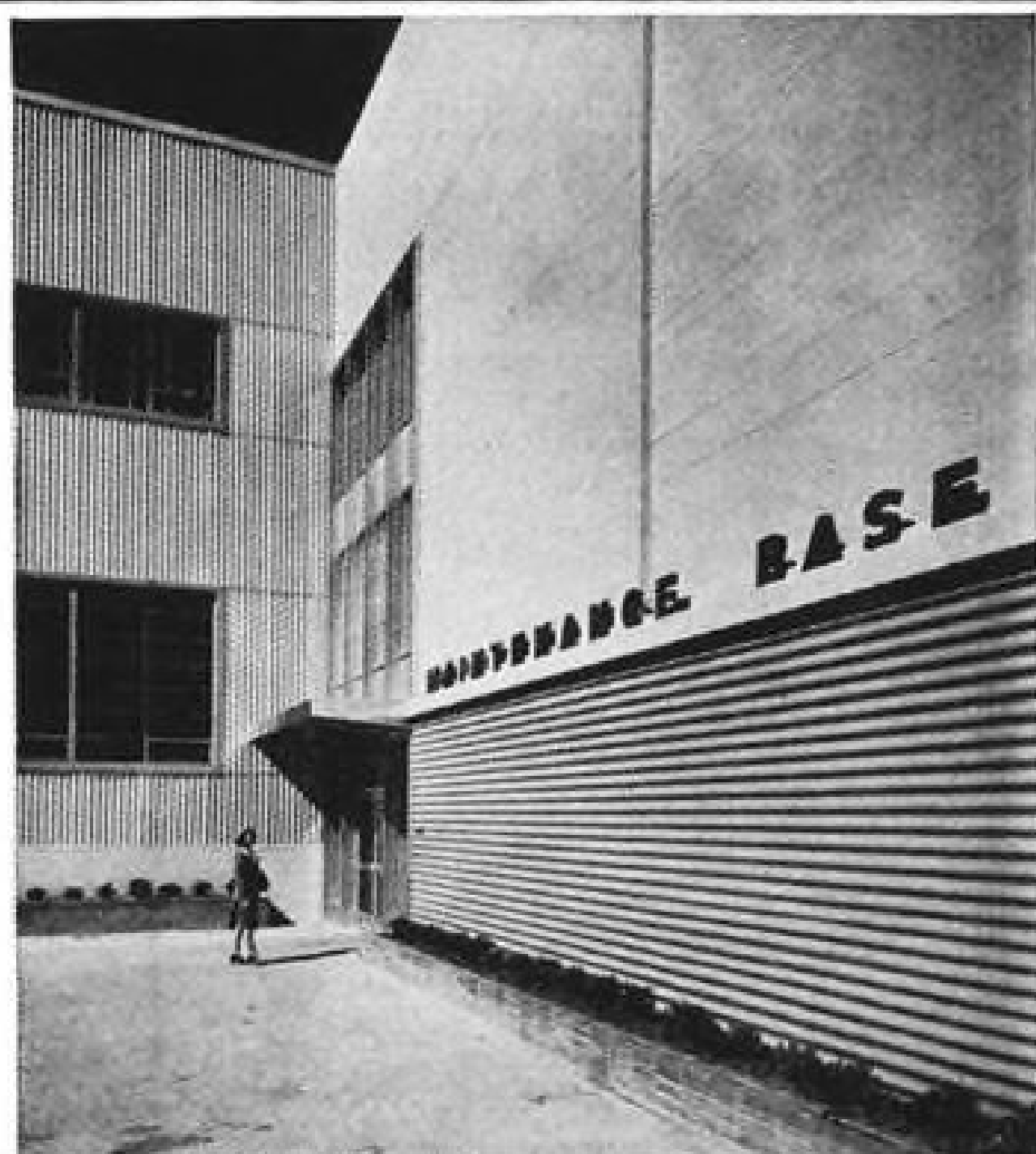
Notice how the strength-building corrugations of Transite are utilized as an element of streamlined design in this United Airlines maintenance base at San Francisco.
