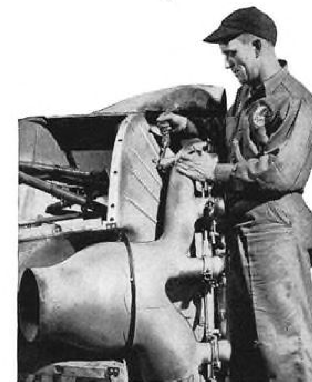
Installing an Inconel exhaust manifold on an engine of a DC-4 operated by Capital Air Lines.
