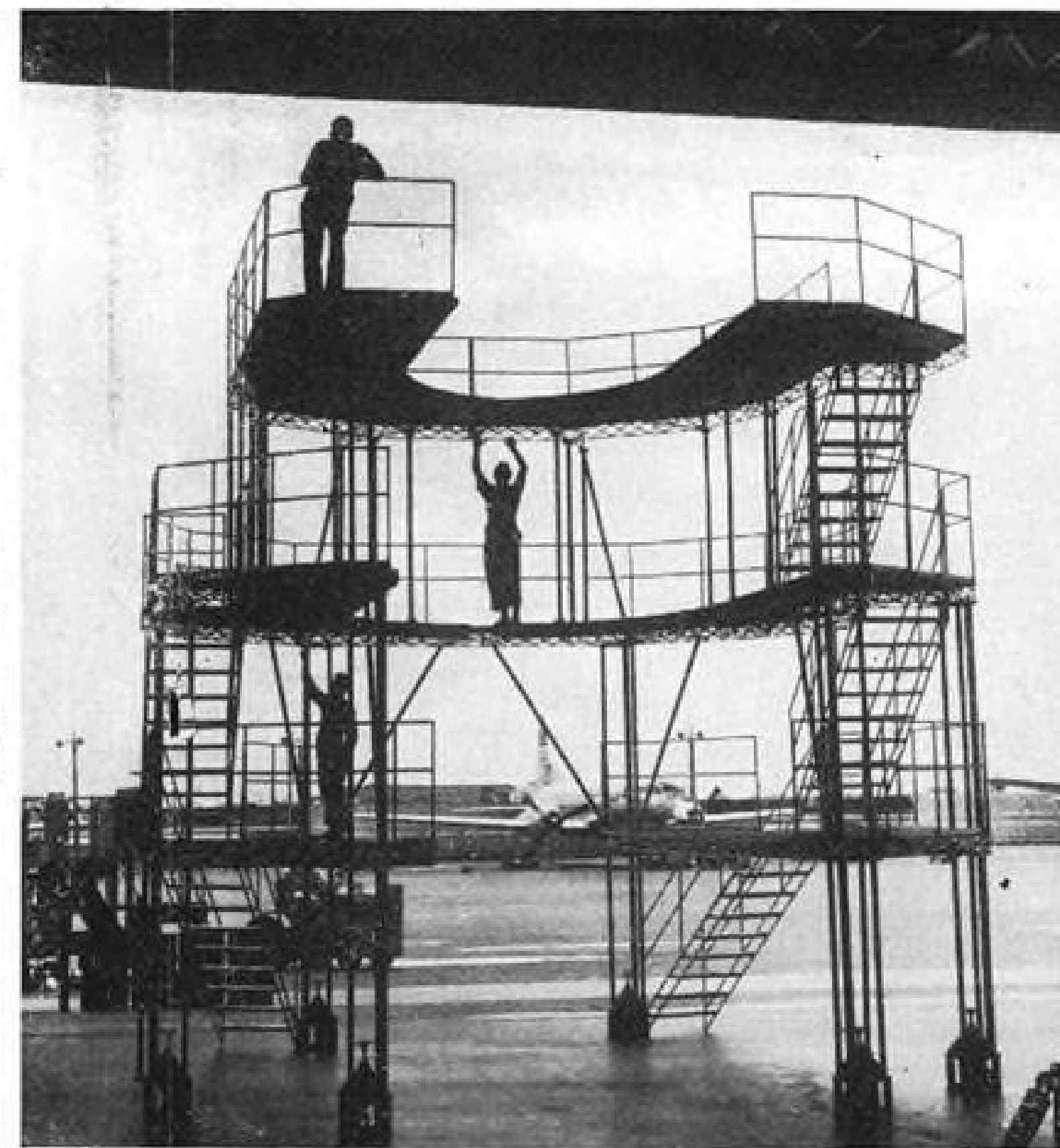
HUGE NOSEDOKK is being readied for giant Stratocruiser. Structure will have electrical, drainage facilities "piped" in.
