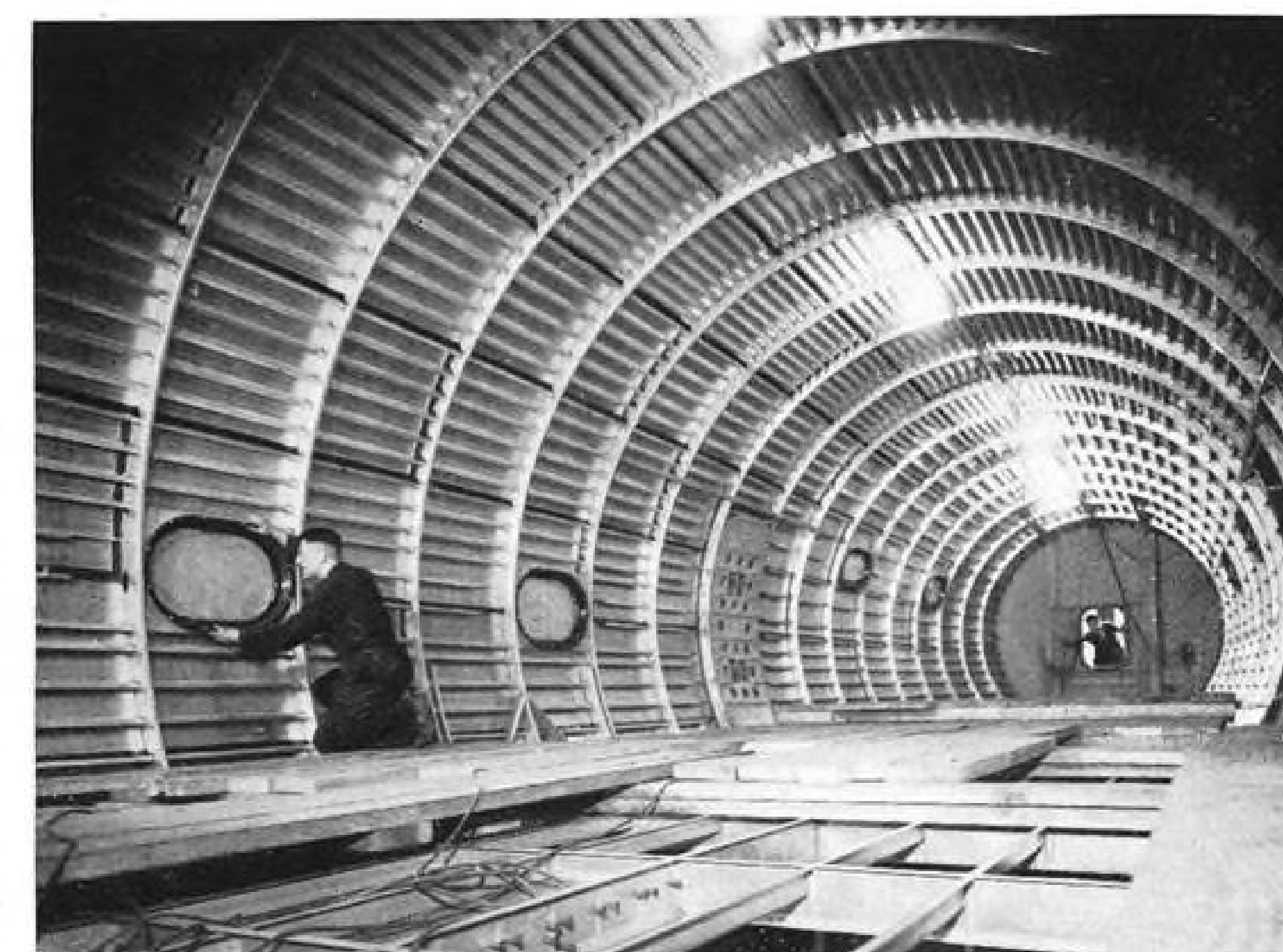
CRAFT'S ROOMINESS is pointed up in this view of rear compartment. Fuselage diameter is 16½ ft. Construction shows conventional belt frame and stringer makeup.
