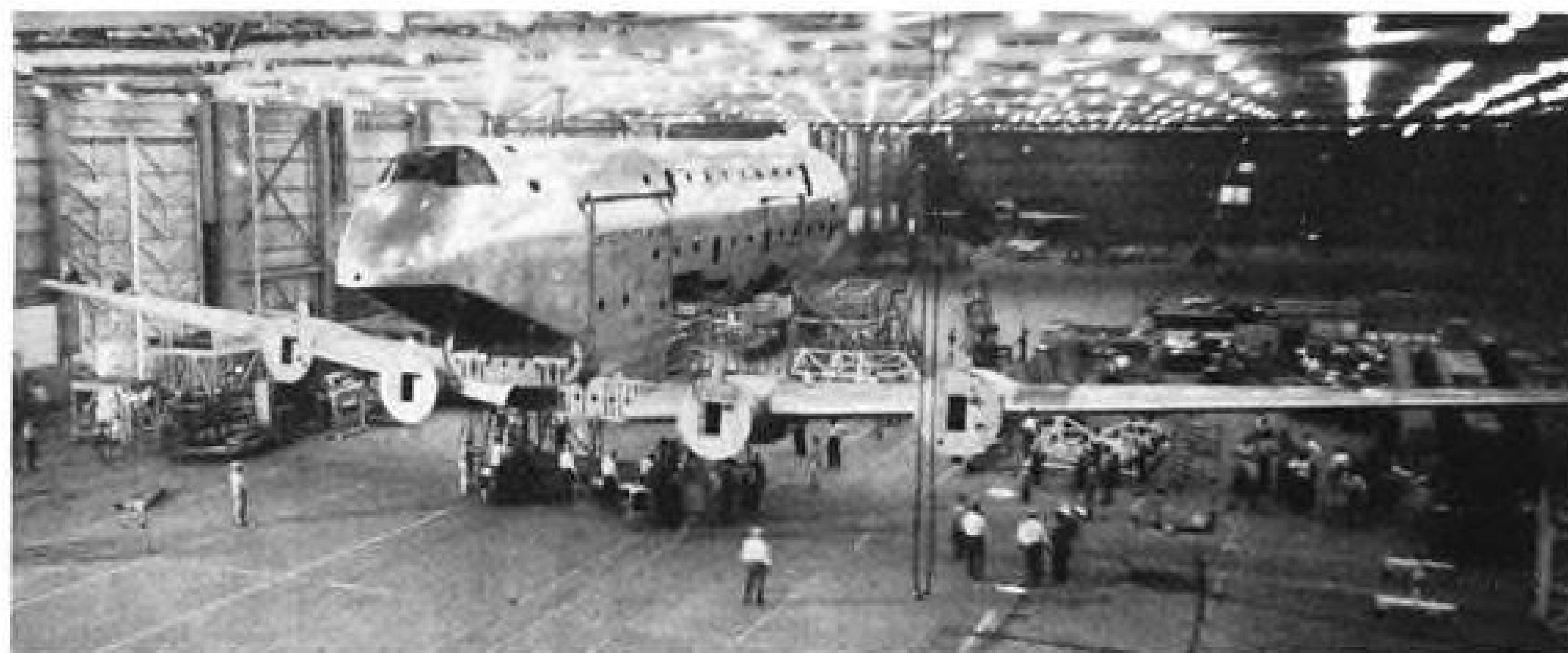
At Douglas Aircraft's Long Beach plant, whale-like 127 ft. fuselage of C-124A is mated . . .
