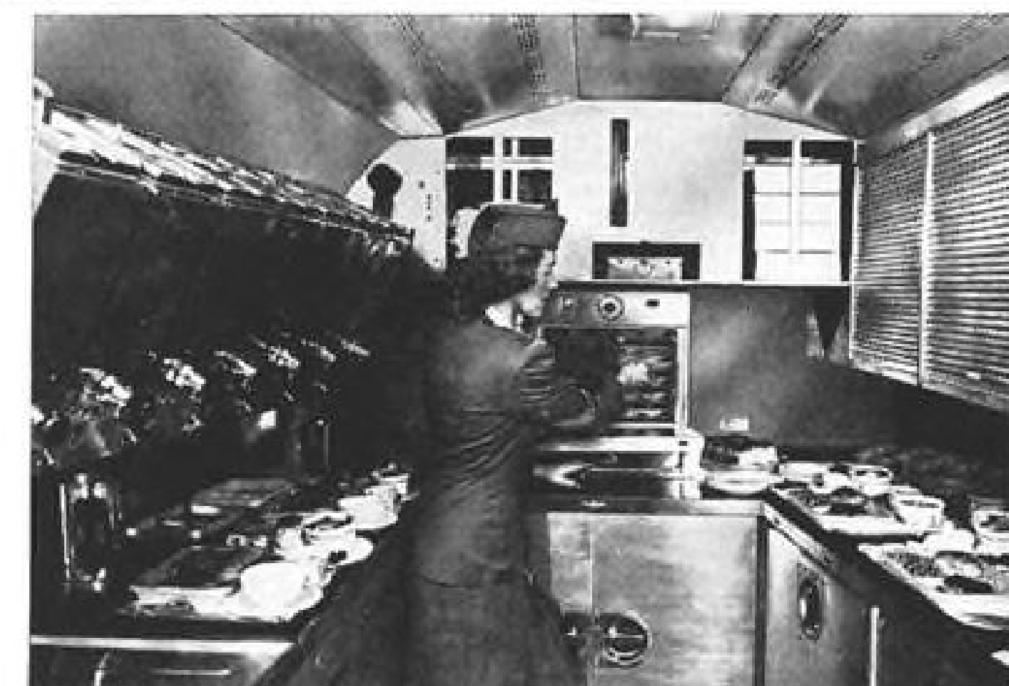
Clean, and easy to keep clean, chromium-nickel stainless steel advances hygienic cleanliness in the Stratocruiser. Its galley can serve 75 persons 3 meals without being restocked.
