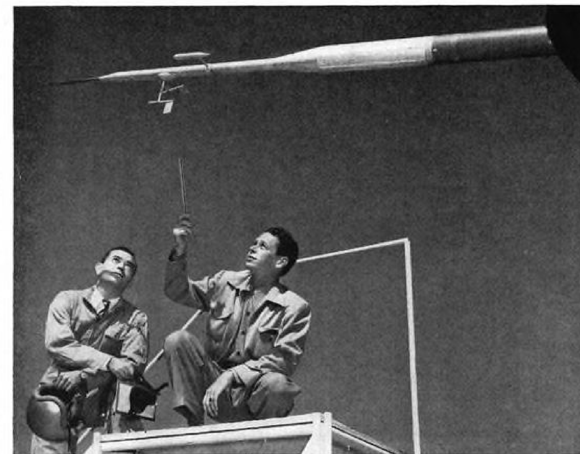
Slender, needle-nose "spear," under test by Northrop Aircraft, is crowded with instruments to give instant telemetered readings of airspeed, yaw, angle of attack, temperature.
