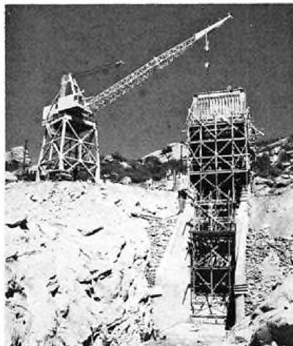
This tower will house motors being tested. Flames will be retained in 75-ft. pit.
