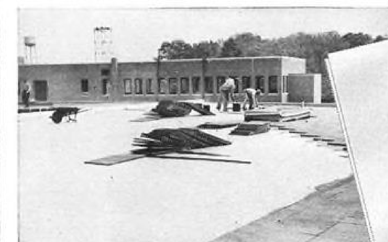
Applied "Ferrobord" offers a smooth, unbroken face, without openings, for easy application of insulation and built-up waterproofing.
