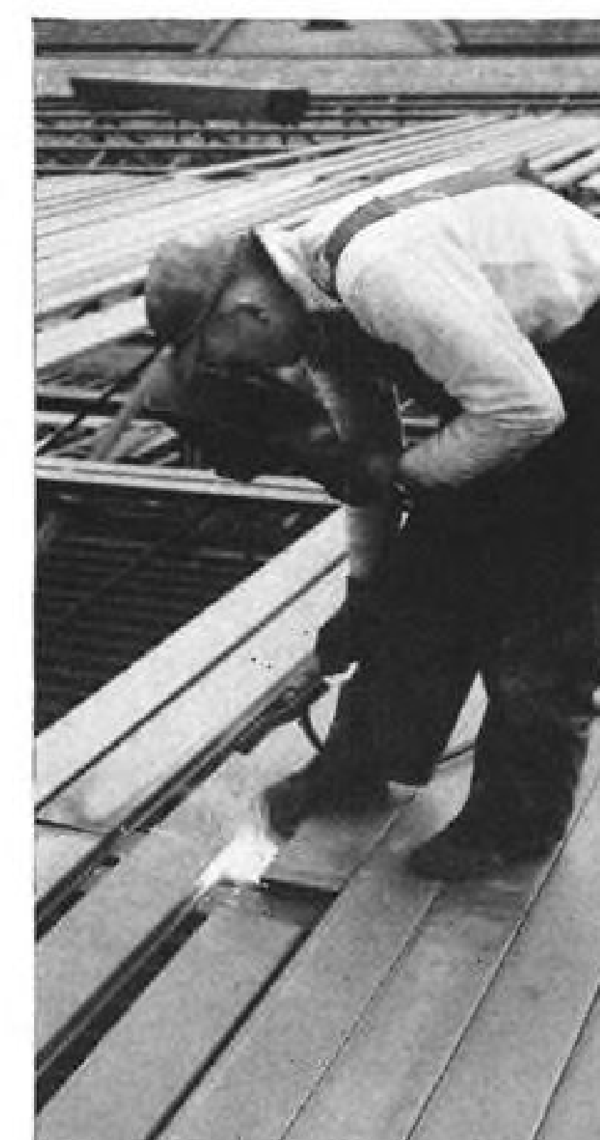
"Ferrobord" can be welded directly to steel units such as Truscon "Clerespan" Joists.
