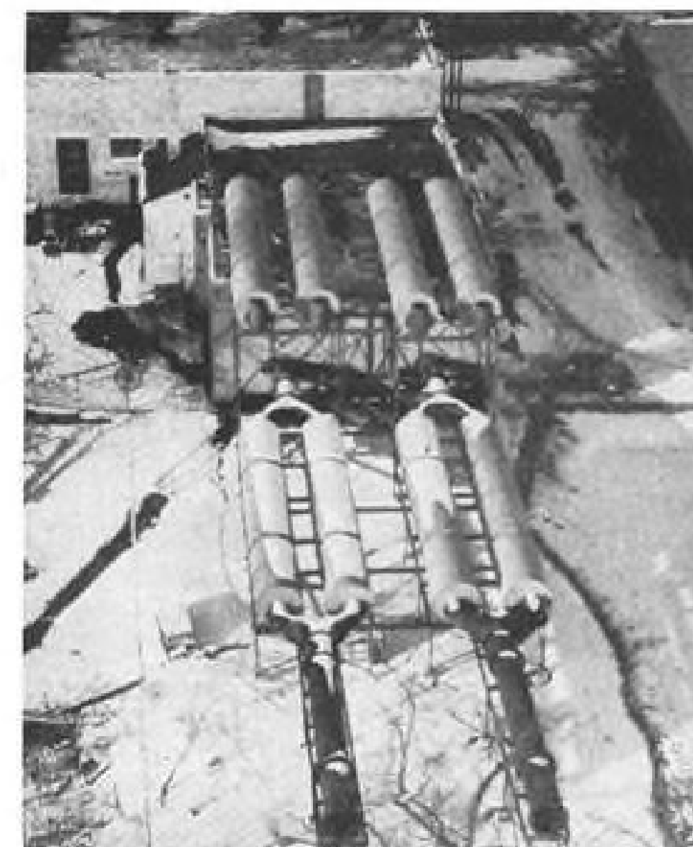
Noise at P&W turbojet compressor test lab is muffled by long tube-like silencers.
