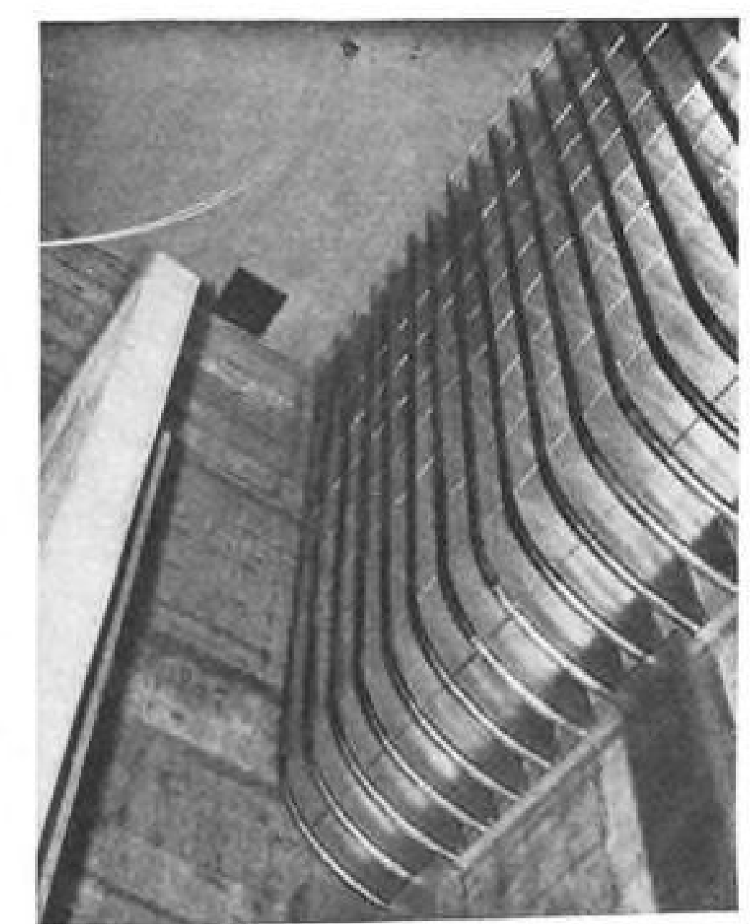
Glass wool in fine-screen metal sheeting reduces sound level in wind tunnel stack.
