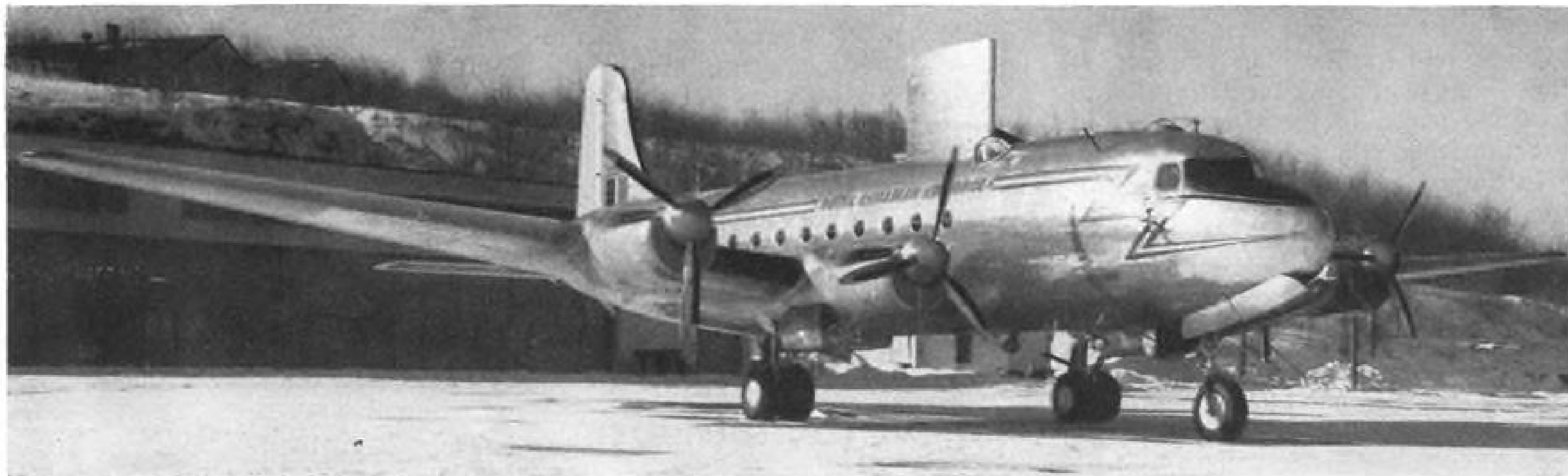
NORTH STAR with fin growing out of its back is used for RCAF icing research. Scientists observe fin in flight, noting icing formation.
