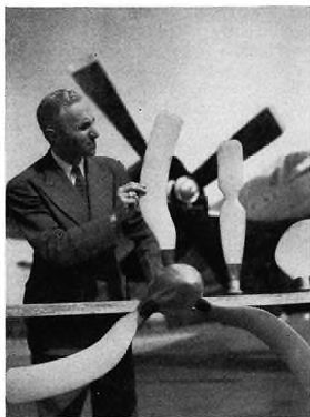
TEST BLADES of Ham Standard assumed many shapes. Left, chief aerodynamicist George Rosen with sweptback blade, one with narrow midsection supposed to ward
