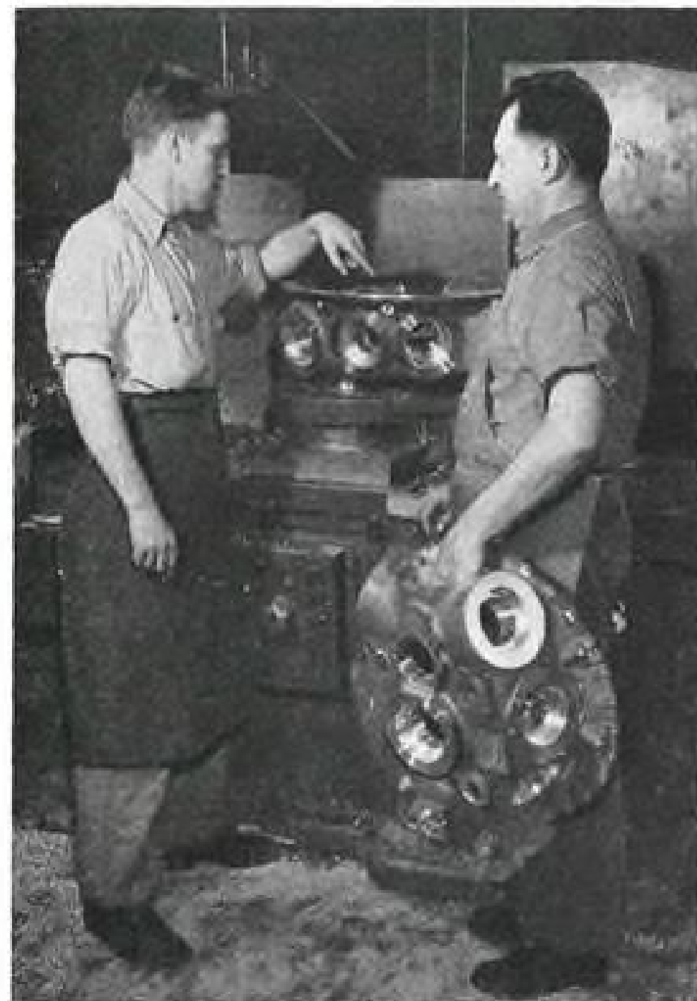
LIGHT WEIGHT Cast magnesium accessory case weighs but 30 lb. and is easily hefted with one hand.
