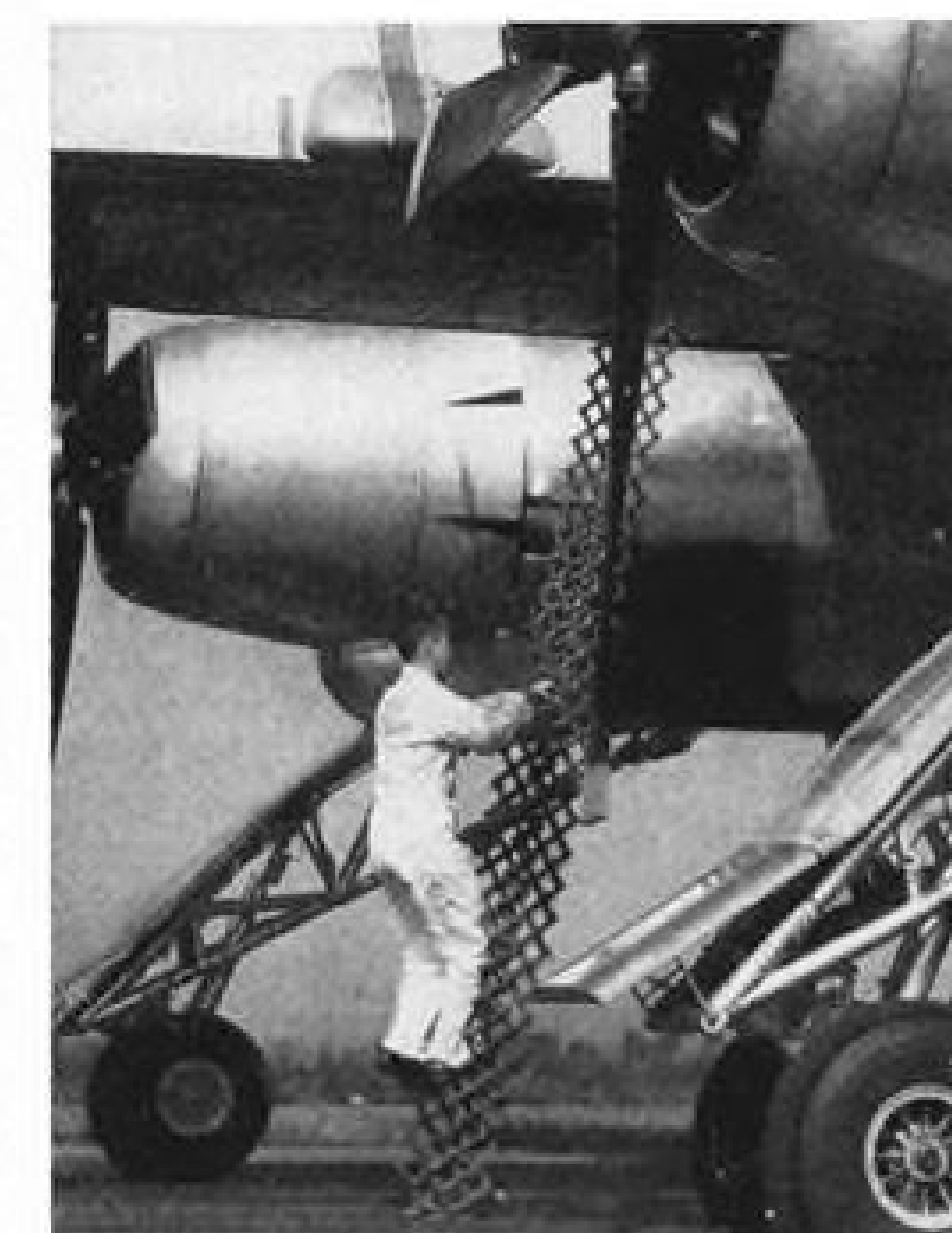
EXTENSIBLE ladder reaches to crew hatch.
