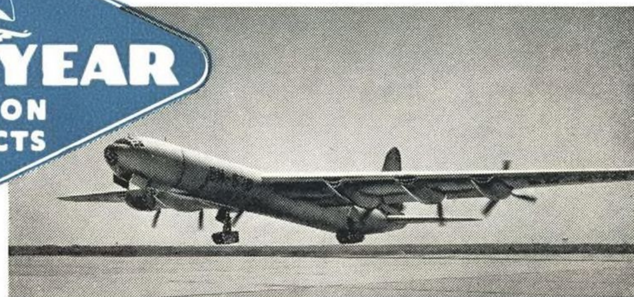
Goodyear track landing gear on B-36
