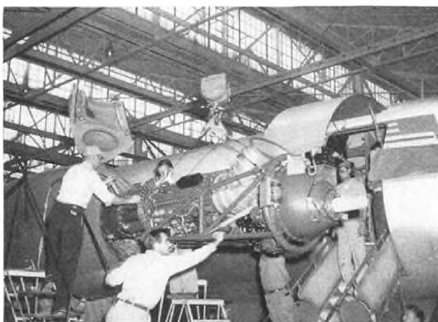
ALLISON 501 turboprop engine. Nacelle contains monorail for . . .
