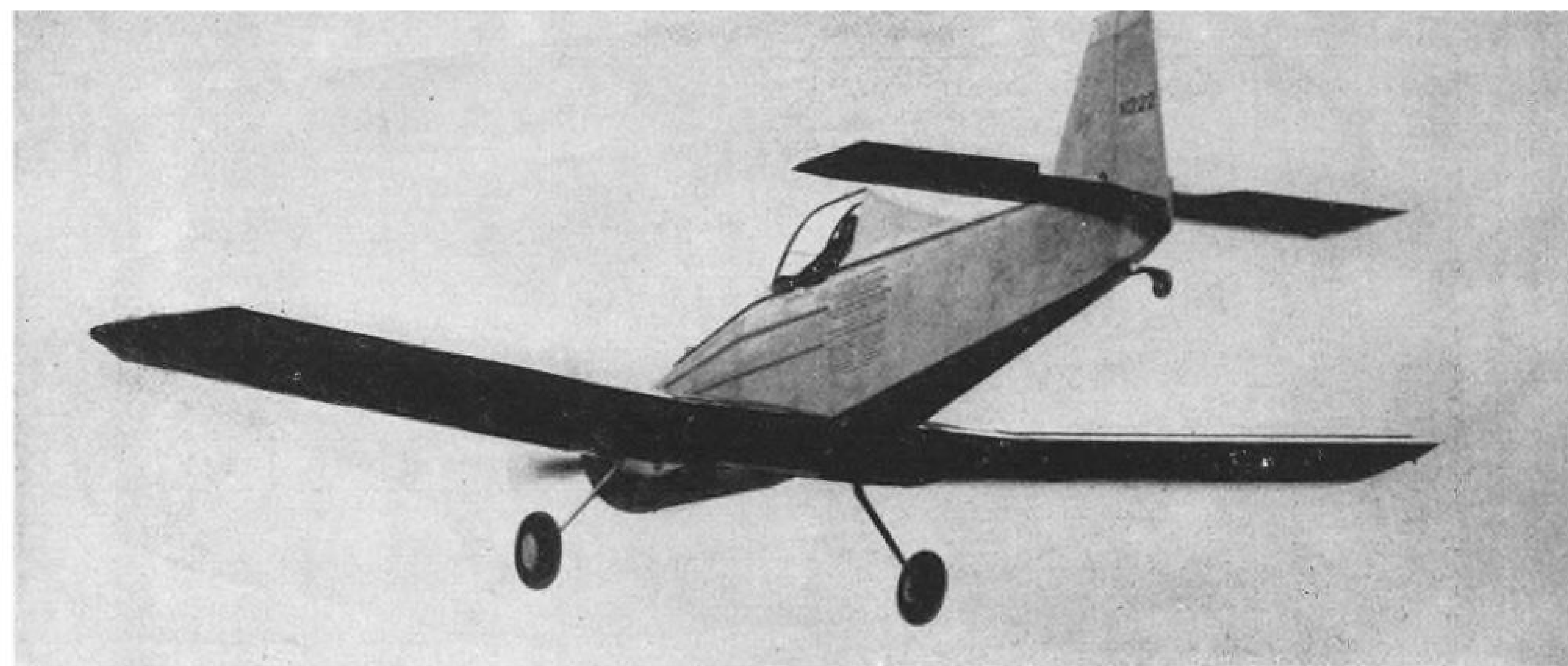
TEXAS A&M TRIES ITS WINGS—Simplified design of new agricultural plane built by Texas A&M's Personal Aircraft Research Center is highlighted in this first-flight-view of the winged sprayer, duster, fertilizer and seeder being piloted by C. W. Von Rosenberg.
