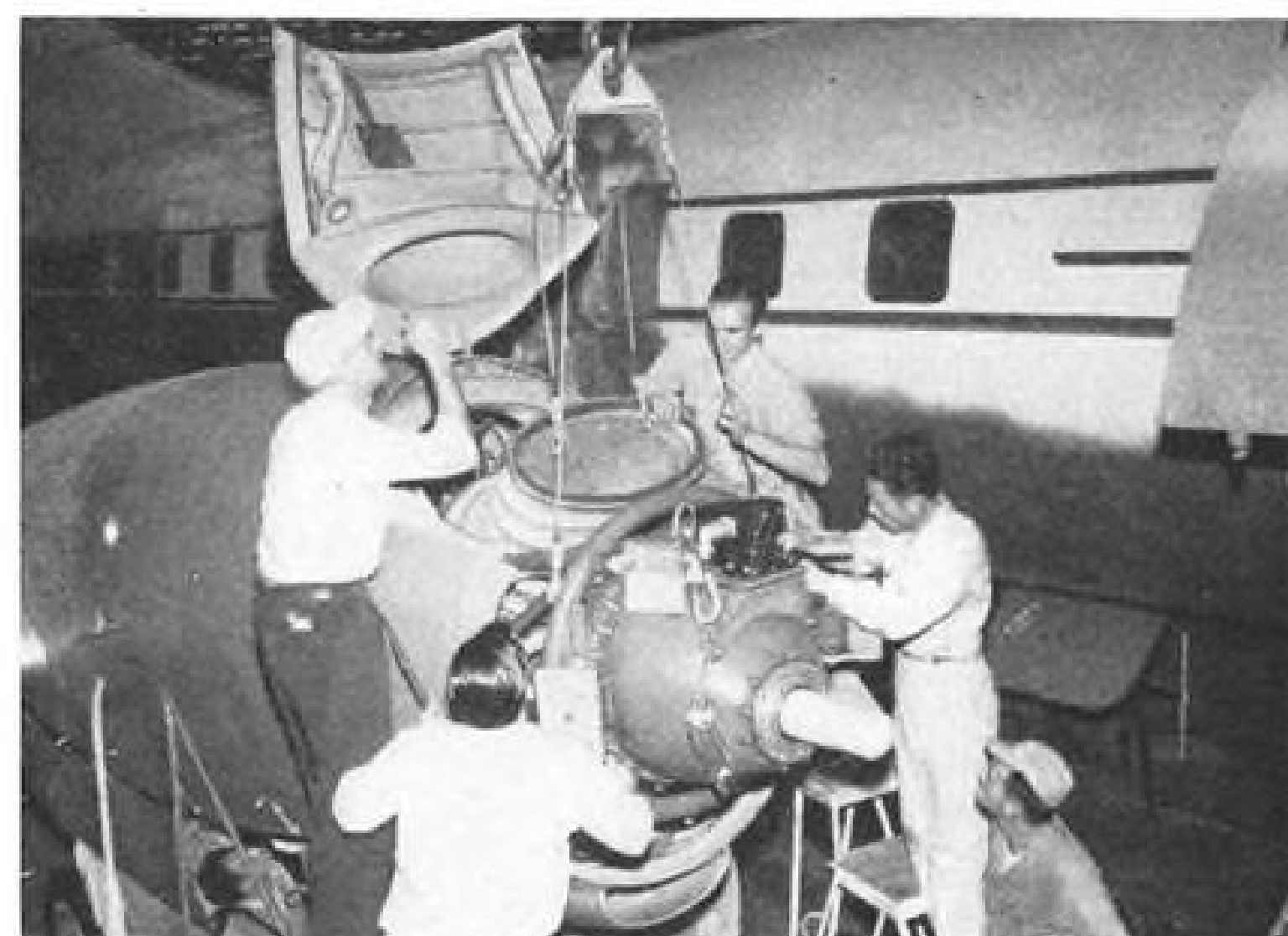
INSTALLATION of 2750-hp. engine. Plane is to fly at year's end.
