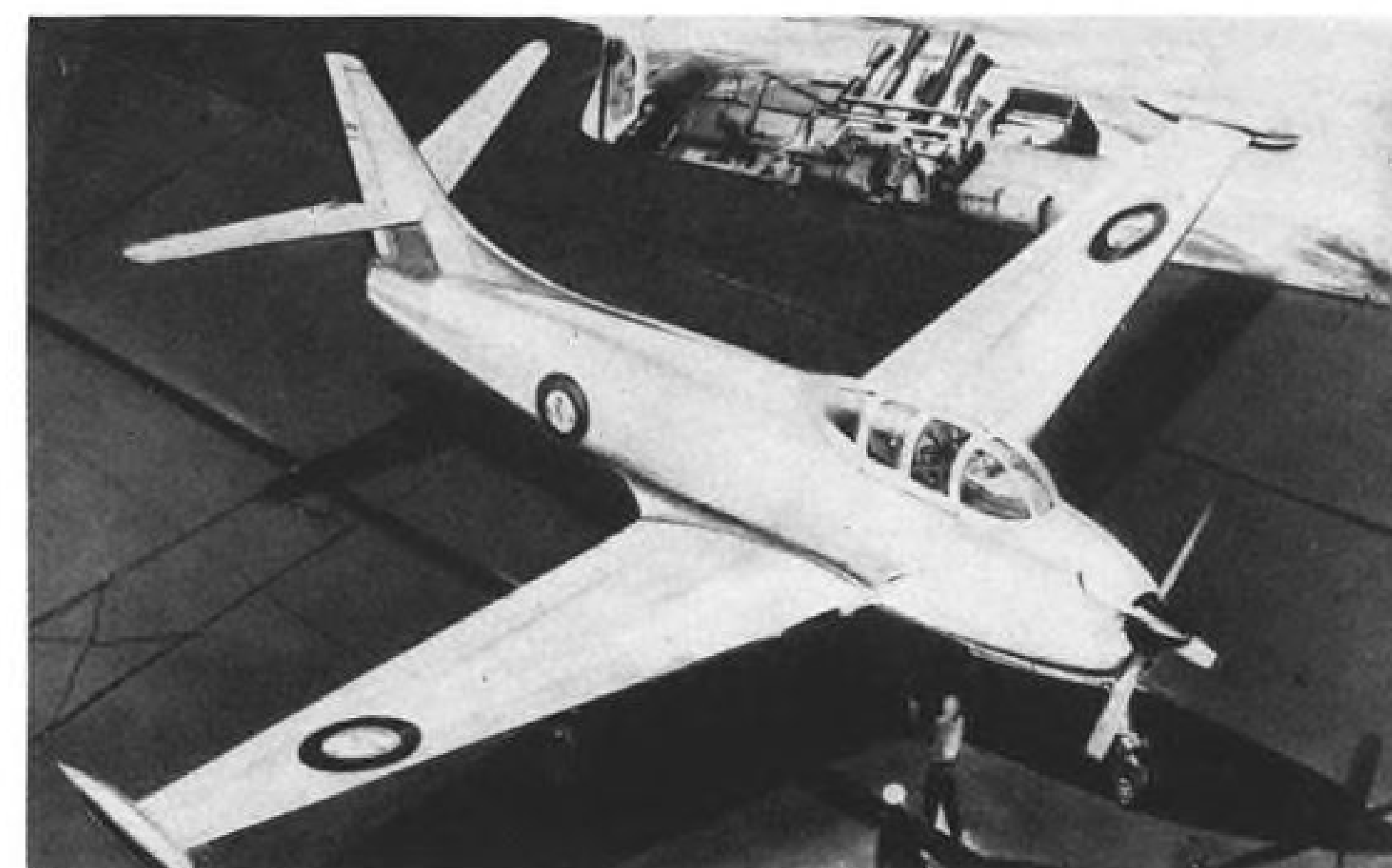
DUTCH JET TRAINER—Nearing completion is the Fokker S.14 2-3 place jet trainer (right) powered by a Rolls Royce Derwent 5 (AVIATION WEEK, Aug. 8, 1949). Sketch shows craft's striking resemblance to Douglas Skystreak. Two occupants sit side by side, third just behind them.
