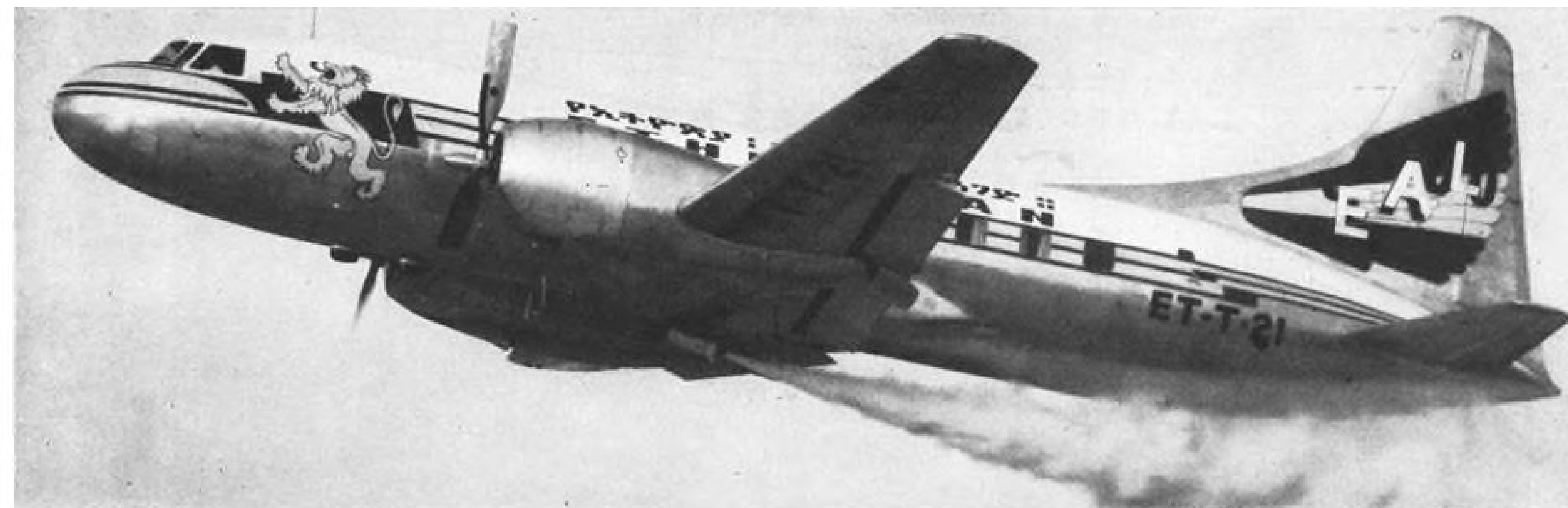
CONVAIR-LINER ROCKETS UP—One of two 41,790-lb. gross 240-s bought by Ethiopian Air Lines shows one-engine take-off (note port prop feathered) using a single Rato bottle. These Convairs have Rato as a standby when operating from high-altitude fields.
